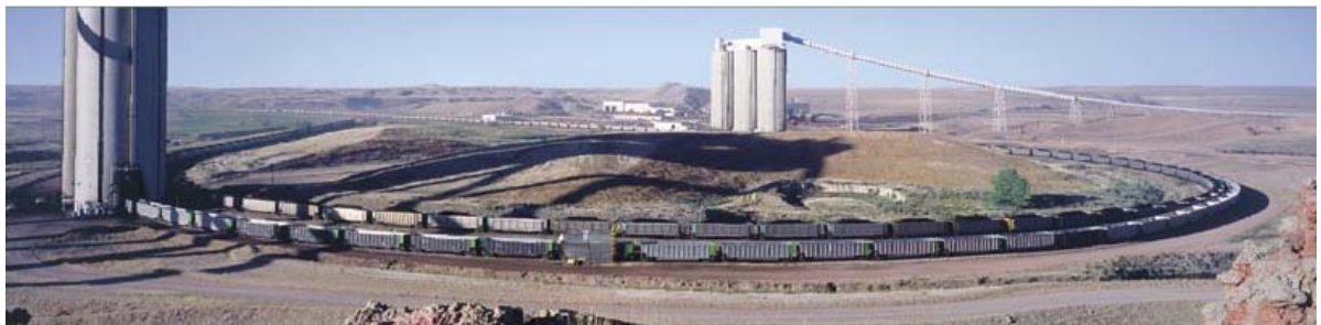
Figure 11: Loading a coal unit train (Peabody Energy, 2006)
