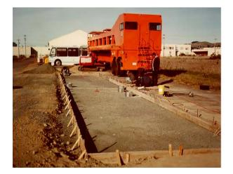
The concrete test sections constructed at the Richmond Field Station (RFS) demonstrated that instrumentation could be successfully embedded in the concrete. The methodologies used to place the instruments were considered adequate given that all gauges functioned correctly throughout the entire test program. The instrumentation and placement methods were developed with help from the US Army Corps of Engineers, Minnesota DOT, and Ohio University.
