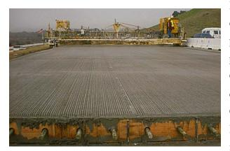
Each aspect of concrete pavement construction was evaluated in terms of paving lane productivity in a preliminary study. In the late 1990s, it had been proposed that the use of Fast-Setting Hydraulic Cement Concrete (FSHCC) was critical to achieving desired construction productivity objectives, and Caltrans was considering requiring the use of FSHCC for lane reconstruction. The following findings are relevant to LLPRS in California:
