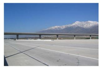
The overall objective of the study was to assess Caltrans long-life pavement rehabilitation strategies for rigid pavements, which aim to add at least 30 years of service life, require minimal maintenance (although zero maintenance is not a stated objective), and allow approximately six lane-kilometers to be rehabilitated or reconstructed within a construction window of 67 hours.
