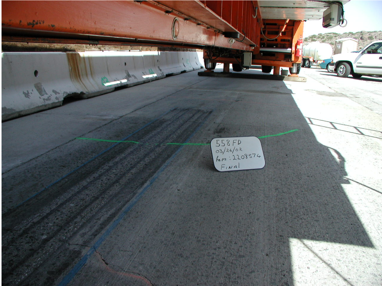
Figure 6.74. Final condition of mid-slab transverse crack and Crack 2 after 2.209 million repetitions.
