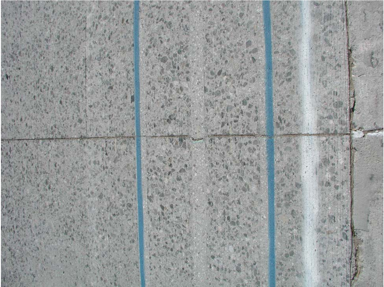
Figure 6.29. HVS Test Section 557FD, Joint 36, prior to HVS testing.
