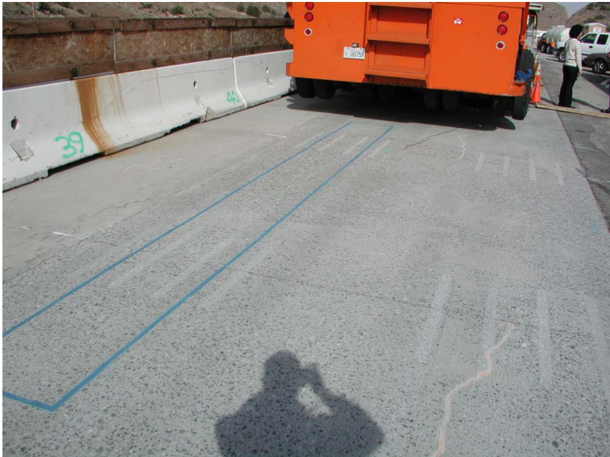
Figure 6.2. HVS Test Section 556FD prior to HVS testing.
