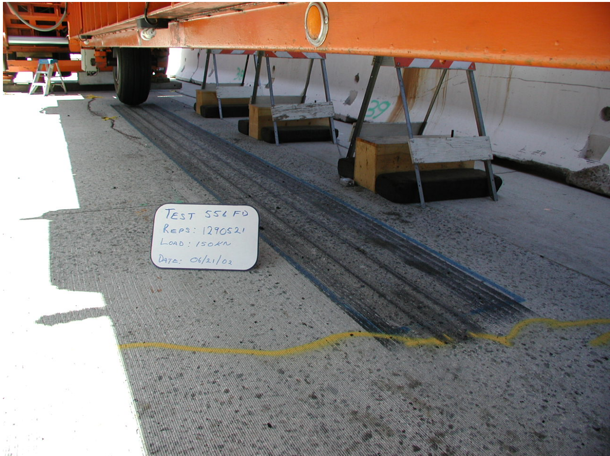
Figure 6.22. Cracking in Slab 40 at end of wheelpath after approximately 1.291 million repetitions.
