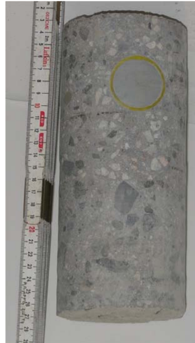
Figure 2.32. Core DBR42NWC with FRP dowel located 62 mm above mid-depth of slab.
