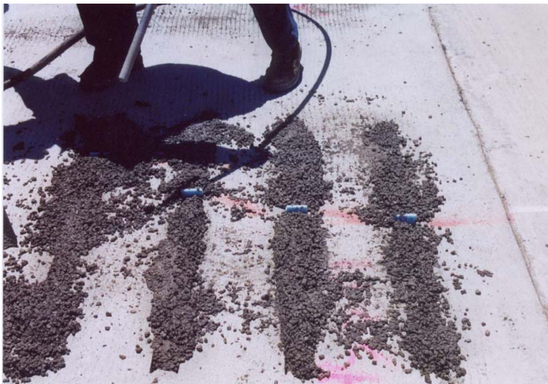
Figure 2.24. Vibration of backfill grout with small stinger.
