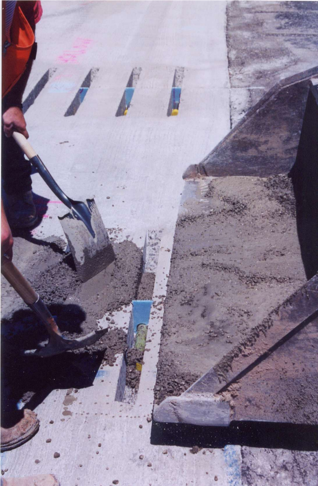
Figure 2.22. Placement of backfill grout in dowel bar slots.
