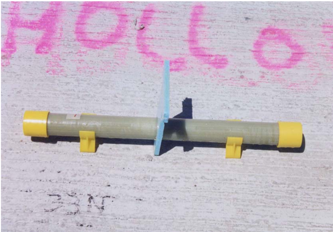
Figure 2.16. Dowel bar retrofit assembly.
