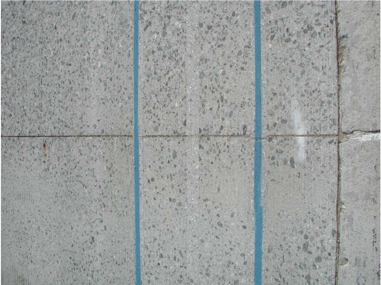
Figure 6.28. HVS Test Section 557FD, Joint 35, prior to HVS testing.
