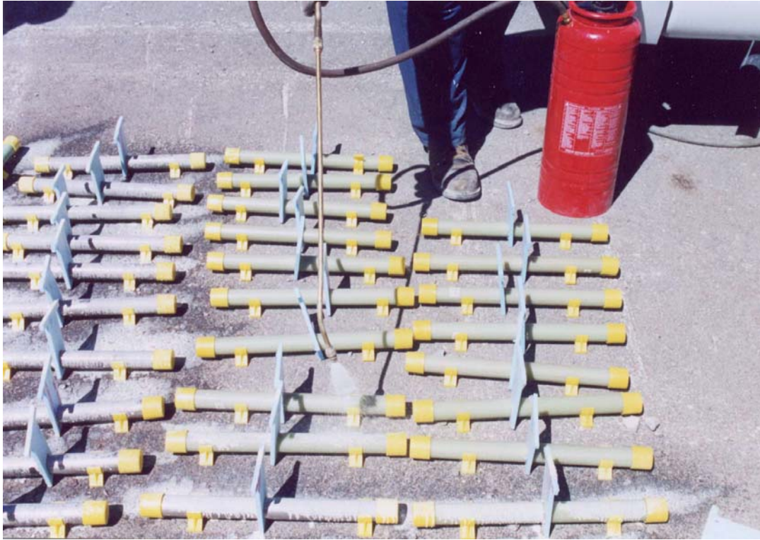
Figure 2.17. Spraying bond-breaker material on dowel bar retrofit assemblies.
