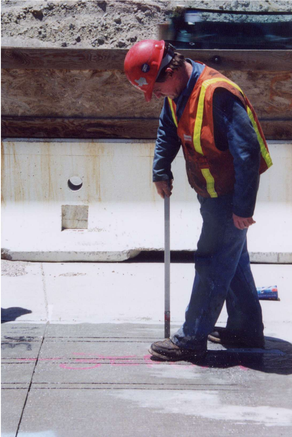
Figure 2.10. Quality control of dowel bar slot cut depth.
