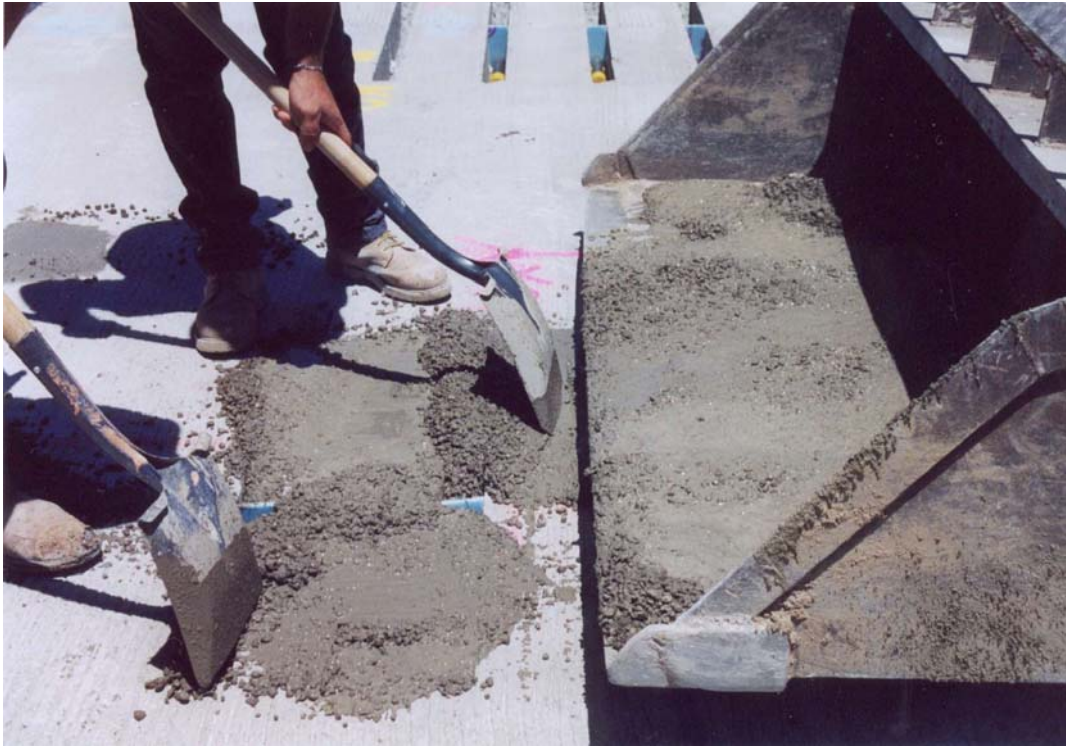
Figure 2.23. Pulling backfill grout into slots with shovels.
