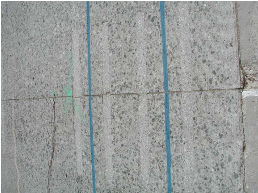
Figure 6.4. HVS Test Section 556FD, Joint 39, prior to HVS testing.
