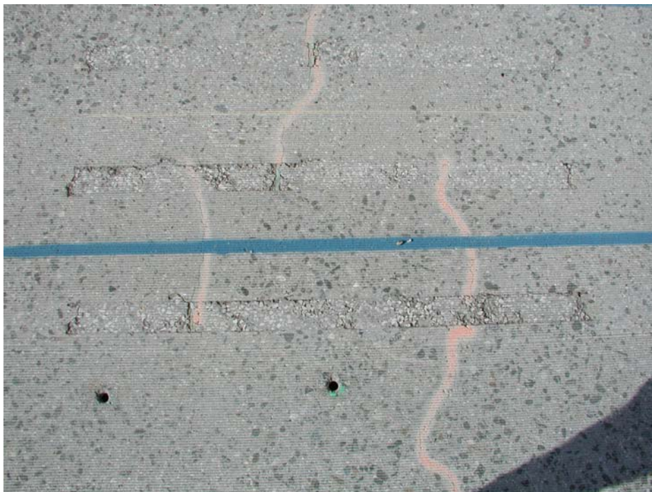
Figure 2.36. Photograph of Crack 1, Section 559FD, in March 2002, showing lack of fines, transverse cracking, and separation at edges.
