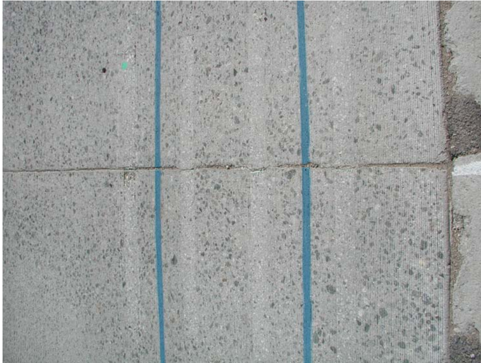
Figure 2.37. Photograph of Joint 33, Section 559FD, in March 2002, showing a small amount of lack of fines and separation at the edges of the dowel slot closest to the slab center.
