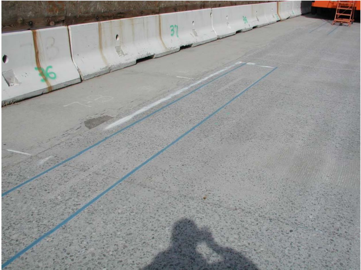
Figure 6.27. HVS Test Section 557FD prior to HVS testing.
