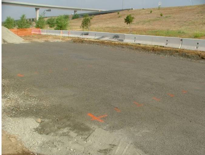
Figure 5. Precise setting out of the corner locations of the pre-cast slabs.
