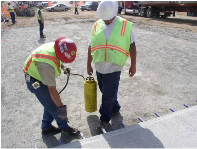
Figure 9. Spraying of the dowel bars with a bond-breaker.
