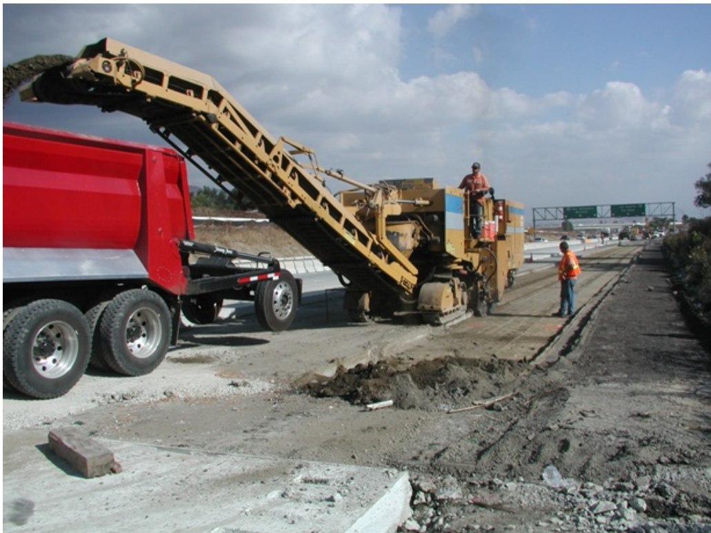
Figure 14: Milling of base.
