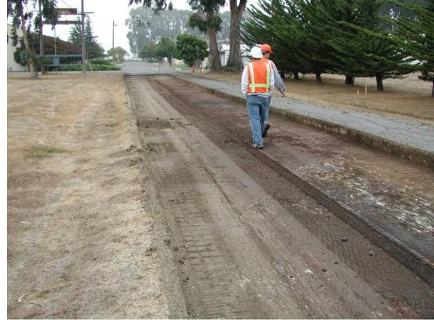
Figure 2.6: Exposed subgrade
