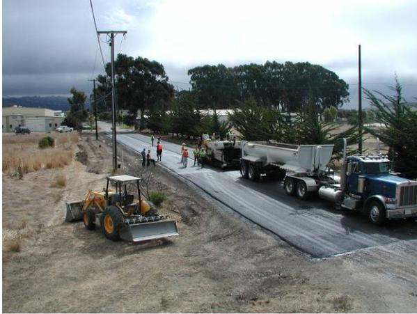
**Figure 2.13: Asphalt concrete placement**
