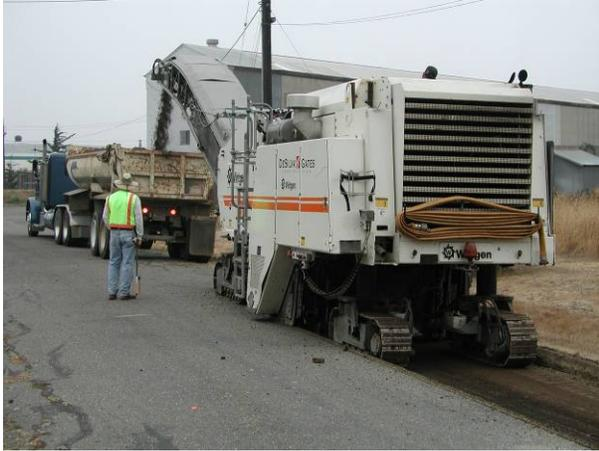
Figure 2.5: Milling of existing roadway
