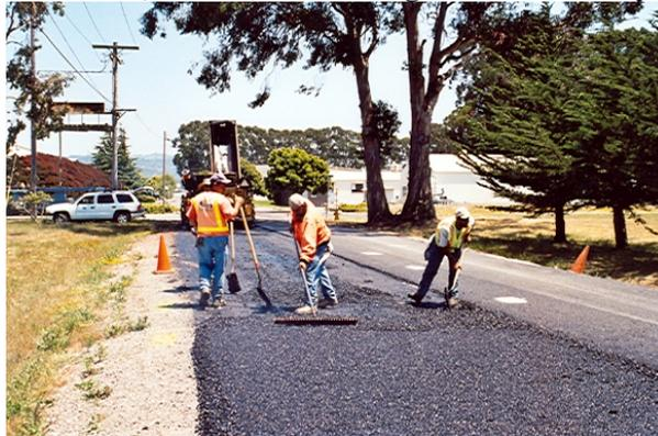
Figure 5.3: Overlay placement (MB4-G).
