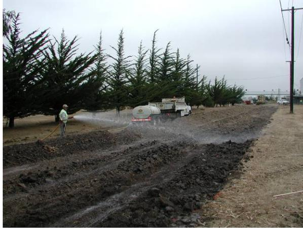
**Figure 2.7: Subgrade preparation**
