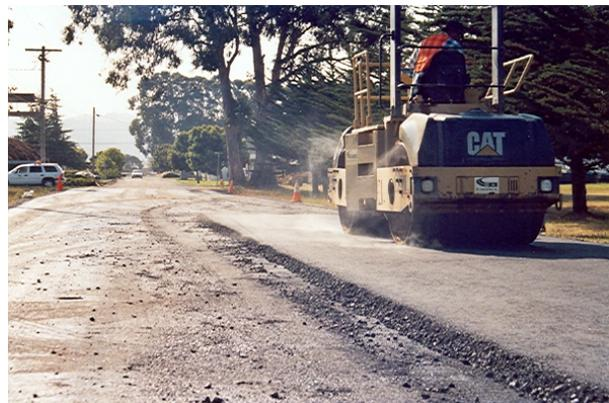
Figure 5.2: Overlay compaction (AR4000-D).
