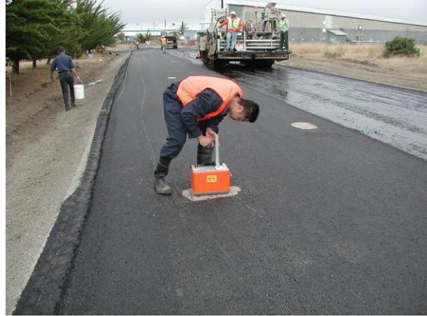
**Figure 2.14: Nuclear density testing**
