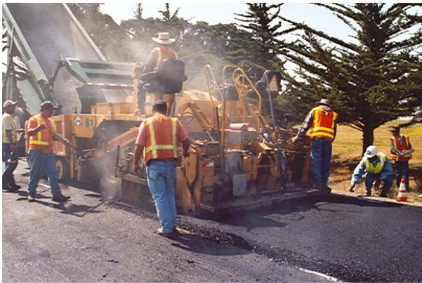
Figure 5.1: Overlay placement (RAC-G).
