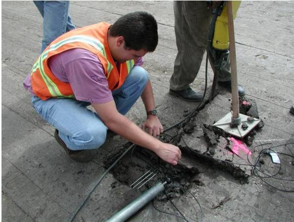
**Figure 2.8: Installation of Time Domain Reflectometer**
