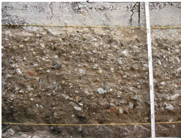
Figure 3.48: 588RF#12 weaker cemented base material.
