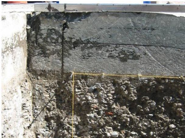
Figure 3.16: 582RF moisture in asphalt concrete layer bonds.
