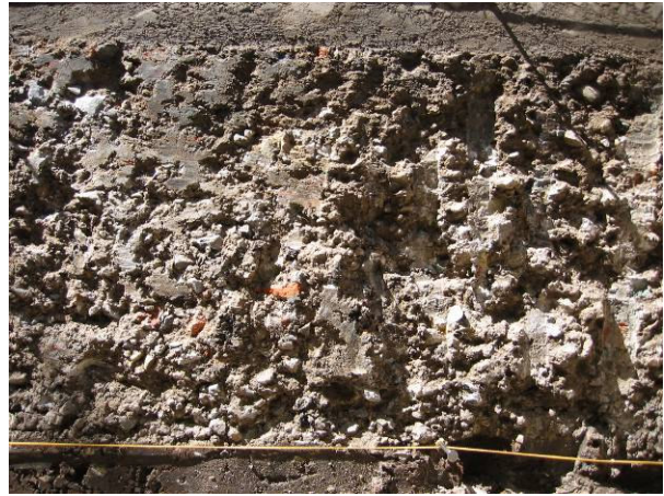
Figure 3.33: 586RF strongly cemented base.
