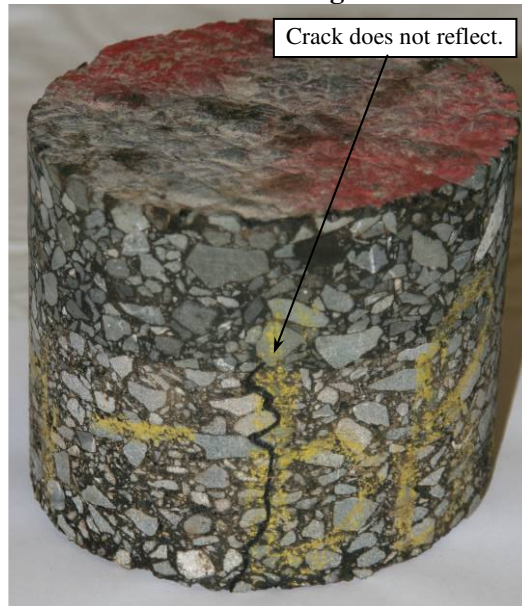
Figure 3.76: MAC15-G: Cracks on core.
