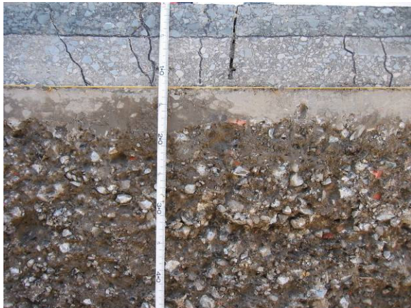
Figure 3.40: 587RF#4 weaker cemented base material.
