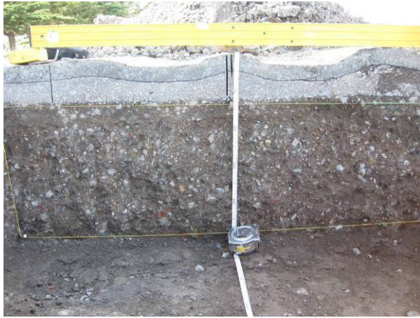
Figure 3.20: 583RF test pit profile. (2)
