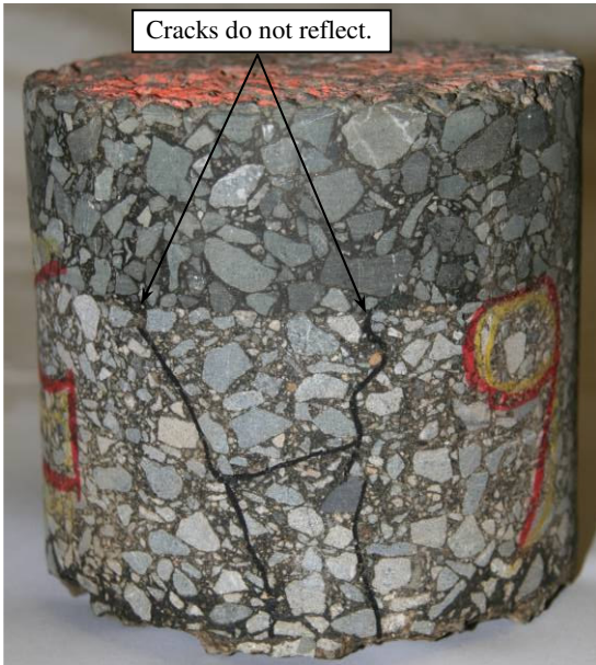
Figure 3.70: MB15-G: Cracks on core.
