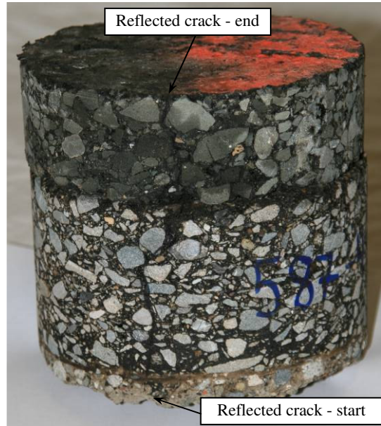
Figure 3.71: RAC-G: Cracks on core.
