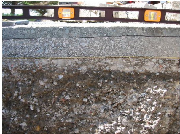
Figure 3.39: 587RF#12 absence of visible cracks.
