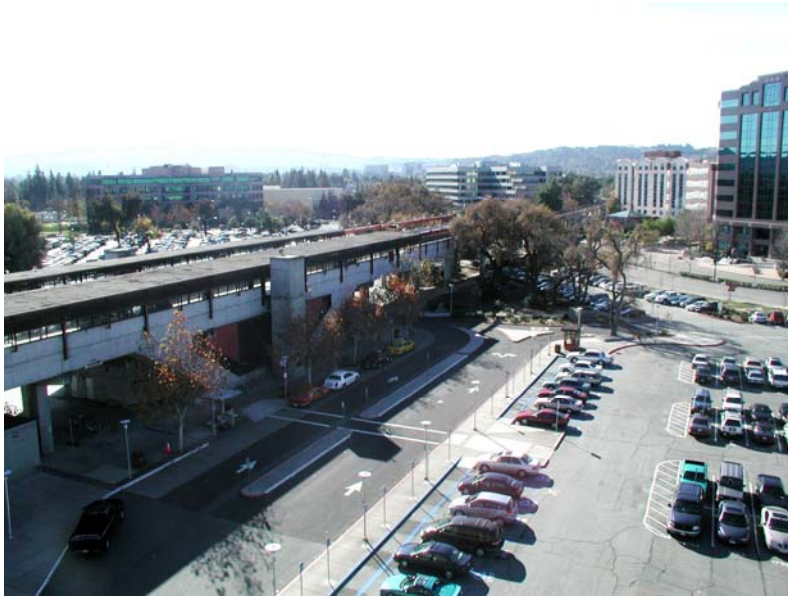
FIGURE 1 Current site conditions, Pleasant Hill BART station.
