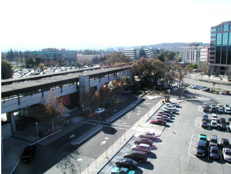
FIGURE 1 Current site conditions, Pleasant Hill BART station.
