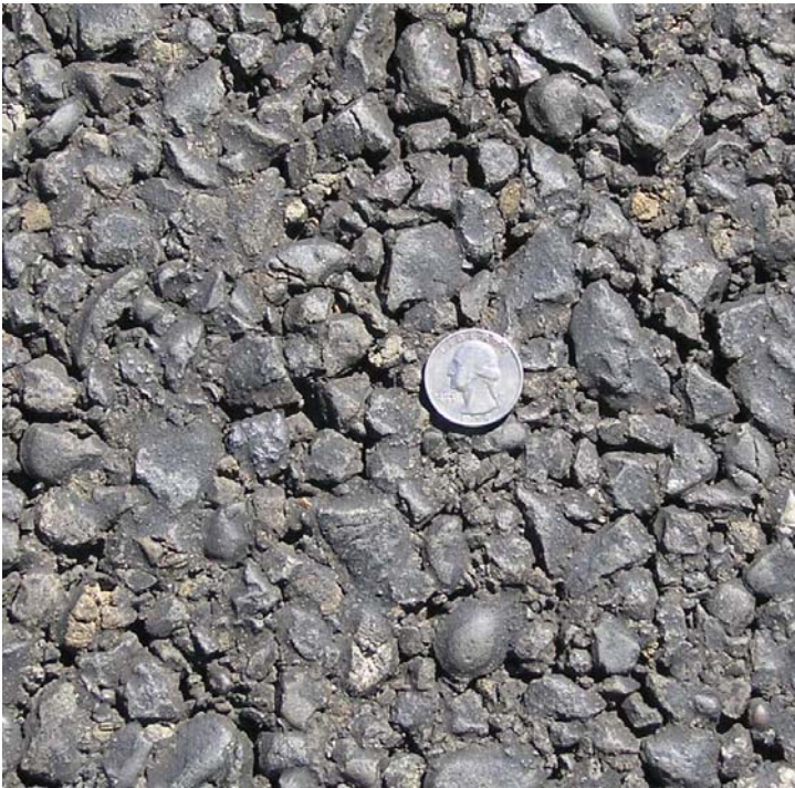
Figure 14: Rubberized open-graded asphalt concrete F-mix (RAC-O F-mix).
