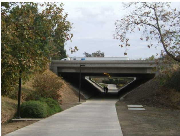
Figure B-7. Interstate 80 Undercrossing in Davis, CA
