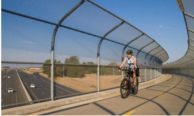
Figure B-6. Highway 50 overcrossing
