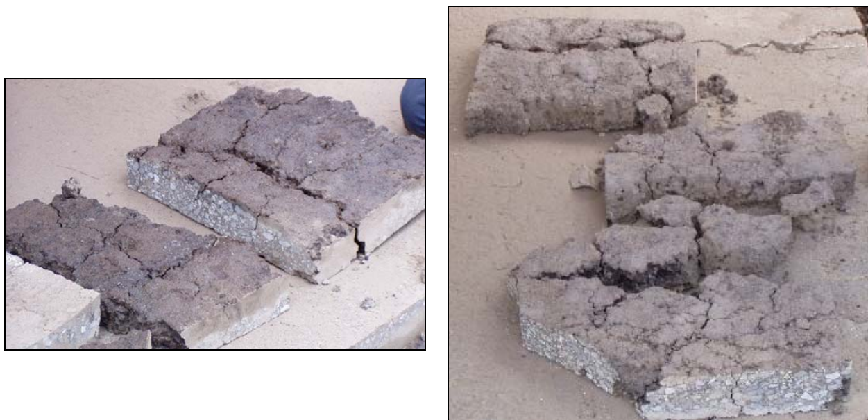
Figure 4.30: Asphalt surfacing from Section 595FD.
