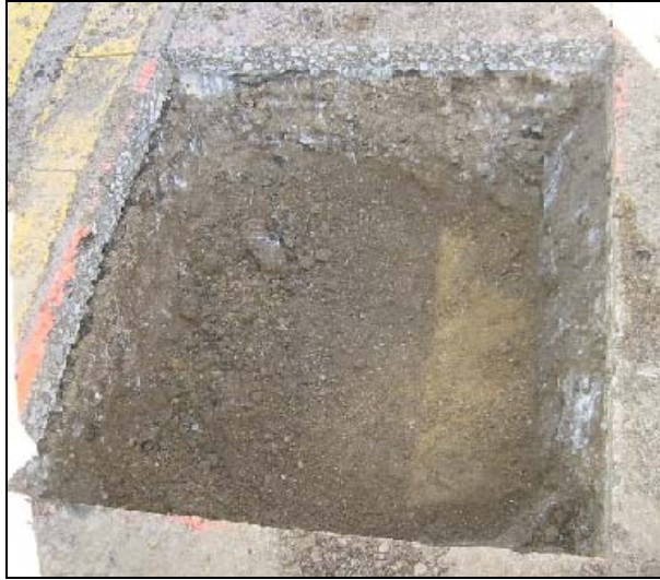
Figure 4.21: Bottom of mainline test pit showing old oil-based pavement.
