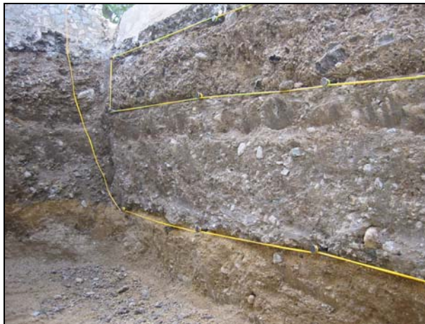
Figure 4.25: Test pit Section 593FD after HVS trafficking.
