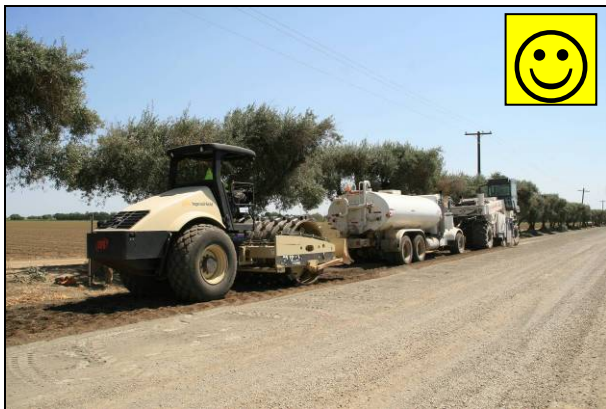
Figure 6.39: Desirable initial compaction procedure.
