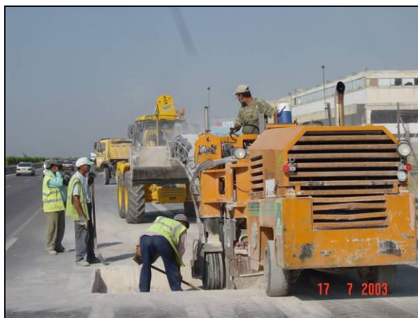
Figure 2.11: Test pit excavation with milling machine.
