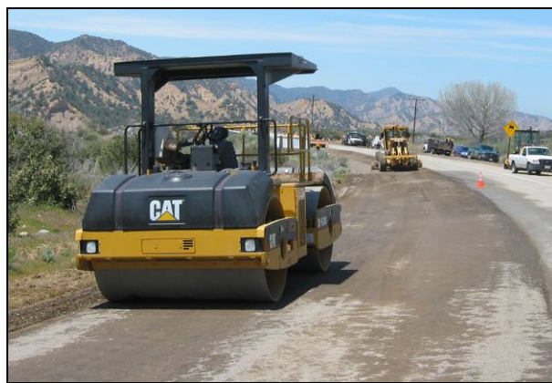
Figure 6.46: Smooth-drum roller behind grader.
