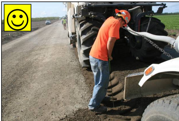
Figure 6.11: Checking recycling depth.
