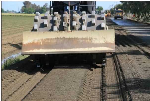
Figure 6.35: First padfoot roller pass.
