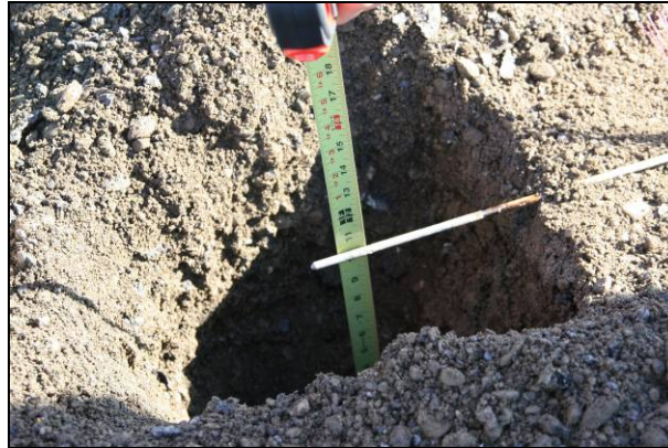
Figure 6.15: Checking recycling depth and grading.
