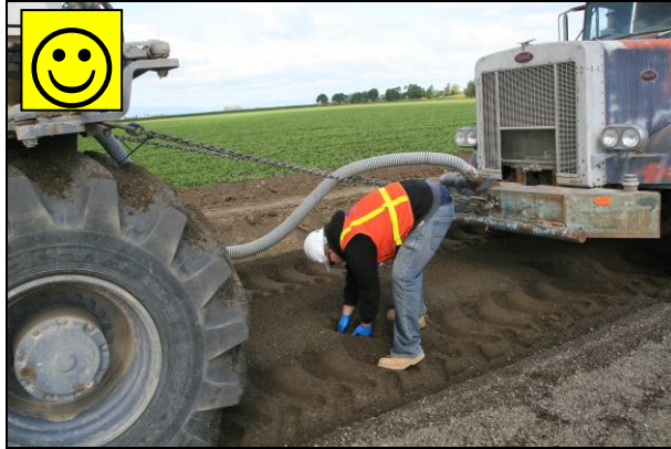
Figure 6.12: Checking material consistency.
