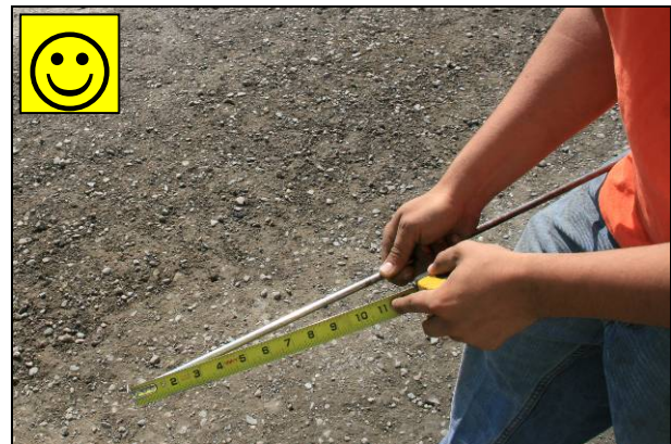
Figure 6.11: Checking recycling depth.
