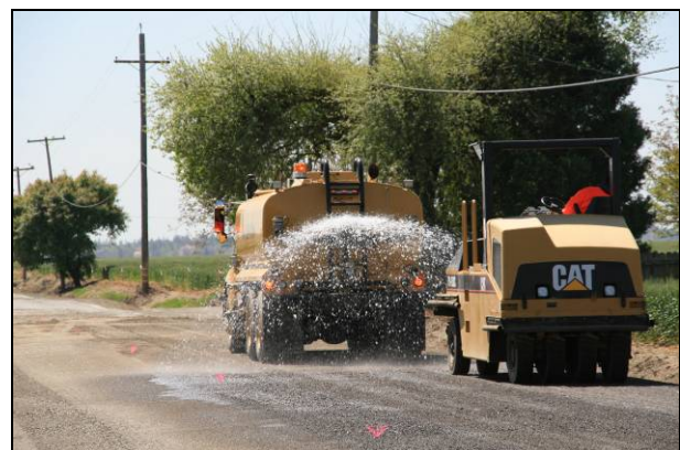
Figure 6.47: Final rolling with pneumatic-tired rollers.
