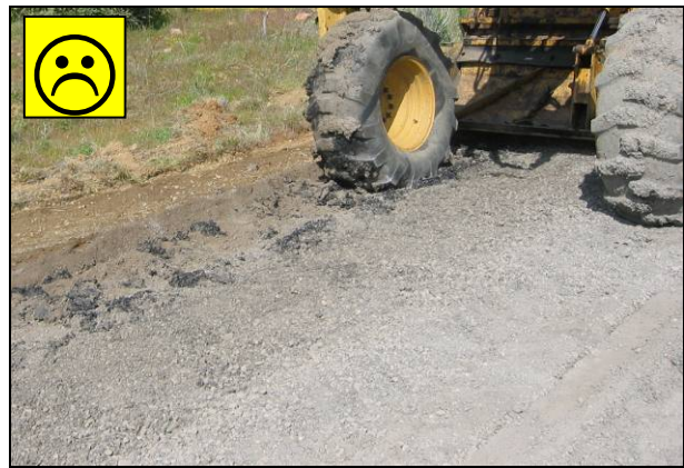
Figure 6.13: Unfoamed binder in recycled material.
