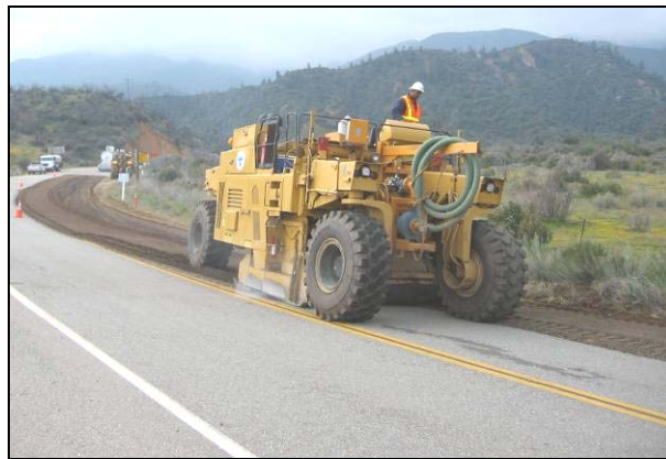
Figure 6.19: Pre-pulverization on FDR-FA project
