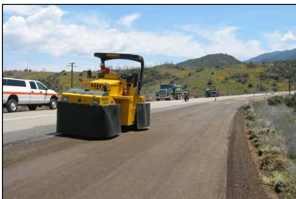
Figure 6.47: Final rolling with pneumatic-tired rollers.
