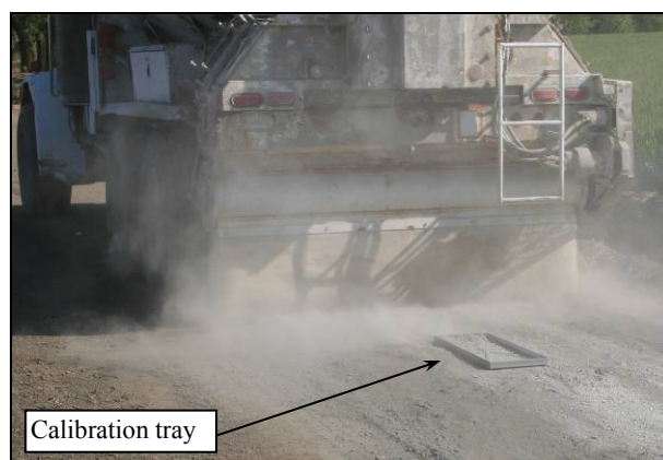
Figure 6.16: Checking active filler spread rate.
