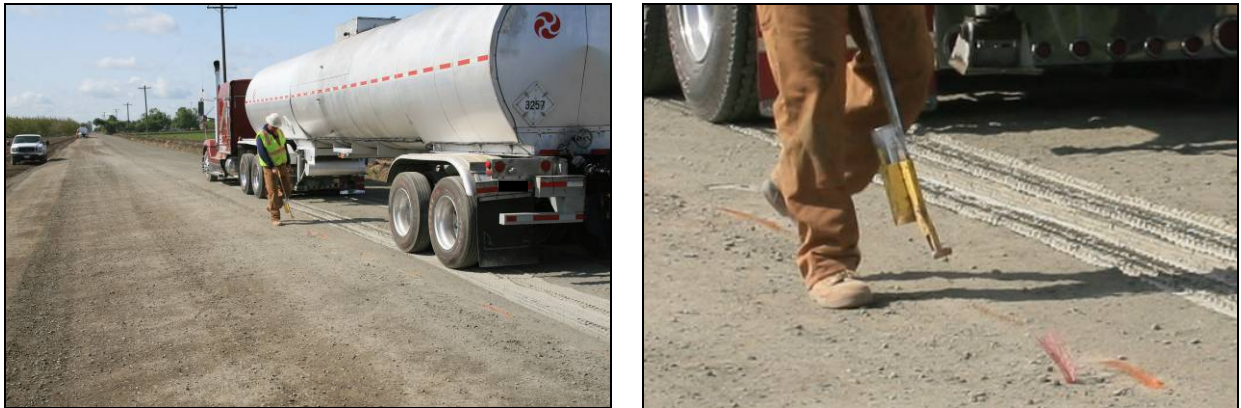
Figure 6.26: Marking directional guides for recycling train.
