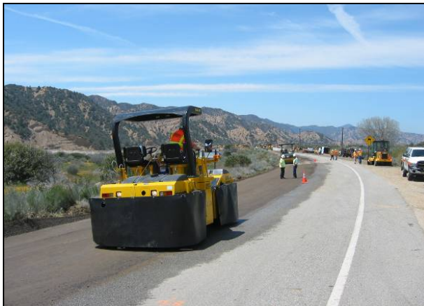
Figure 6.7: Pneumatic-tired roller (PTR).
