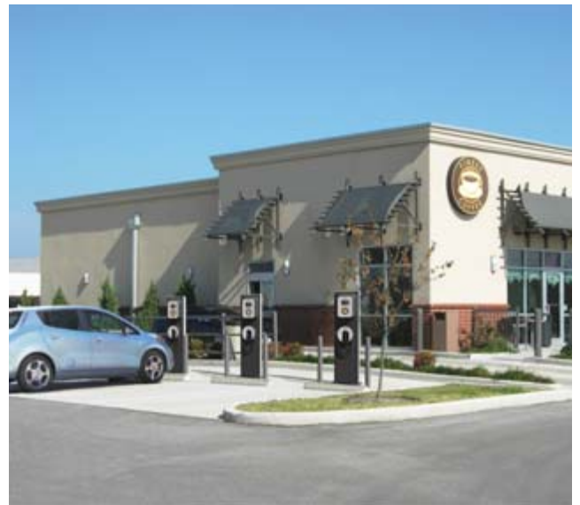
Public charging stations, such as these Blink Level 2 charging stations by ECOtality, will come to retail locations
