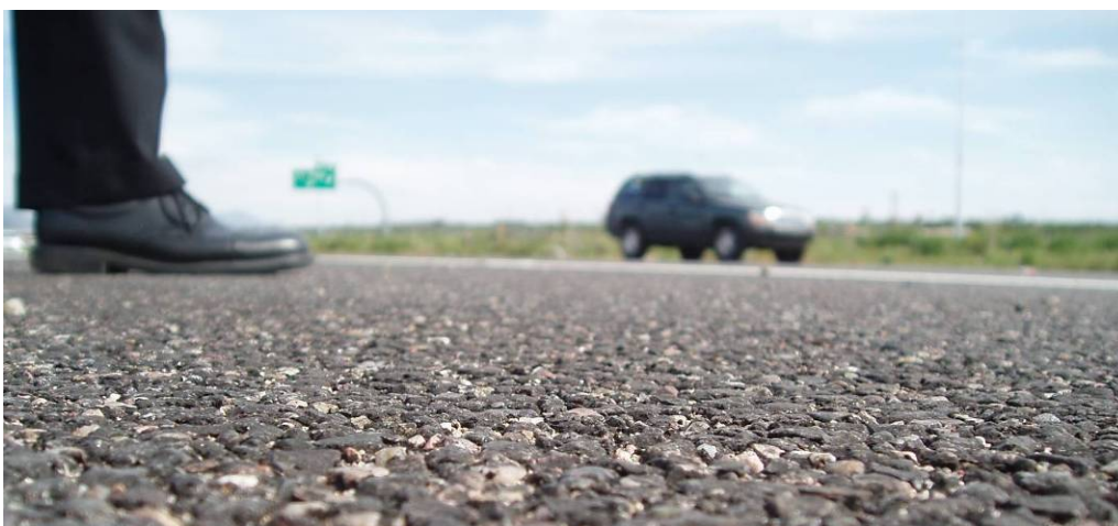
Figure 1.9. Road with Asphalt Rubber Friction Course (ARFC) in Phoenix Arizona.
