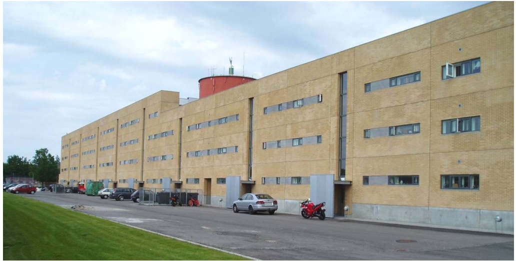
Figure 7.4. New three and four storey apartment buildings constructed close to a highway with high noise levels. At the façade facing the noise, the windows are small and highly noise insulated. The apartments are planned so that secondary rooms like bathrooms, corridors, storage rooms, etc are adjacent to the noisy façade. Bedrooms and living rooms are adjacent to the silent façade.
