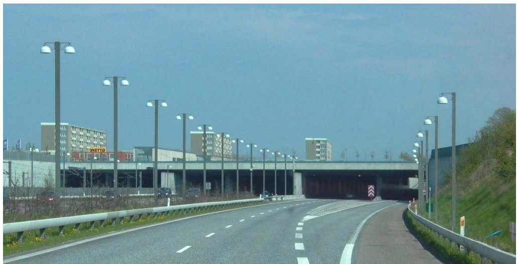
Figure 4.5. 700 m long section of the new highway to Copenhagen airport, Denmark was constructed as a cut and cover strategy in order to reduce the noise exposure for some nearby multi-storey apartment buildings.
