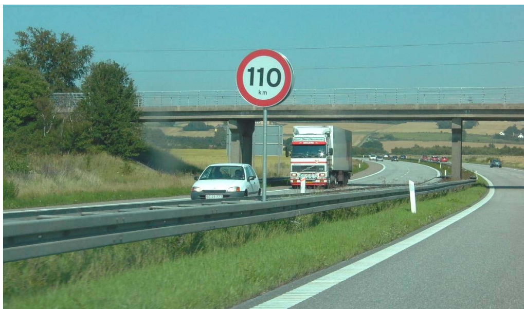
Figure 6.12. Reducing the speed where a highway passes noise sensitive areas could reduce the noise. A solution where the reduced speed limit is only effective in the evening and night period could be considered in order to reduce noise annoyance when people are sleeping. This measure is only effective at reducing noise only if the speed is actually reduced.
