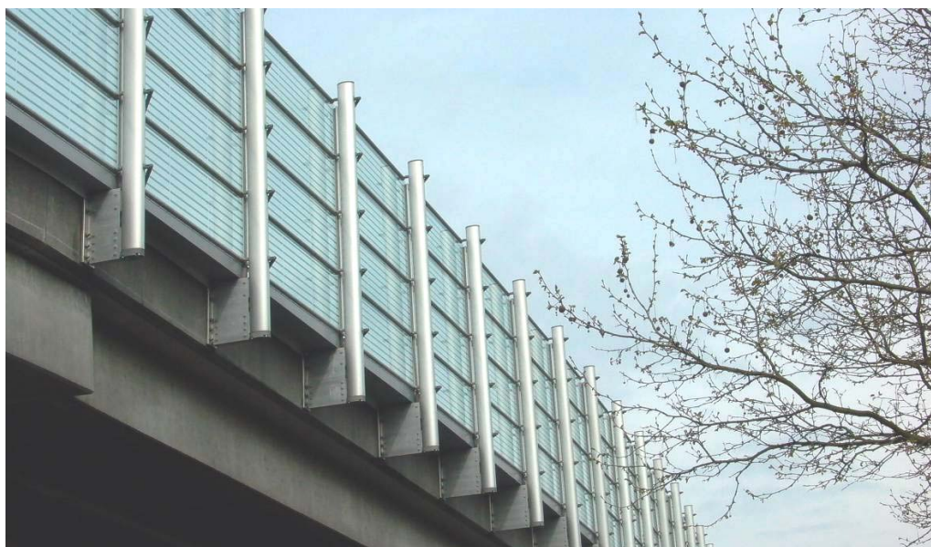
Figure 6.3. Elevated highway through a densely built up urban area in Frederiksberg/Copenhagen with five to six storey apartment buildings. Transparent noise barriers have been used in combination with façade insulation.
