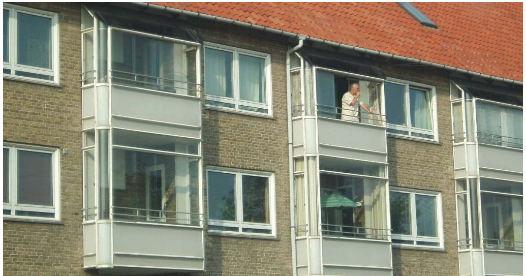
Figure 4.7. Close up photo of glass covered balconies. It is possible for the residents to open up the balconies.
