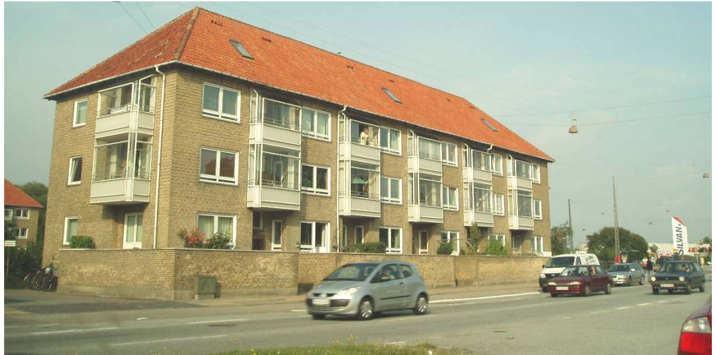
Figure 4.6. Noise insulation of an apartment building by applying glass to cover the façade of the balconies.
