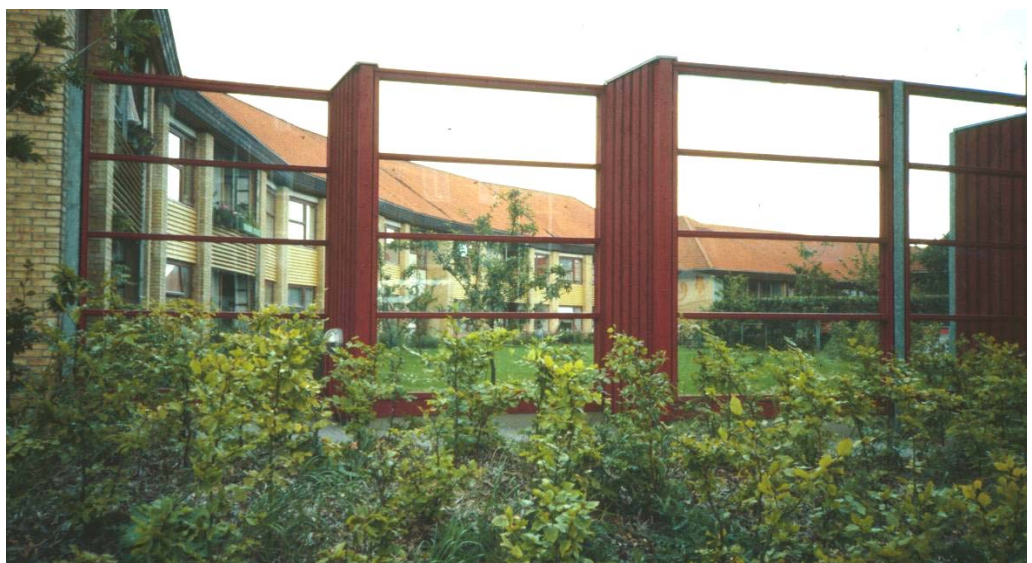
Figure 7.3. New residential apartment building for elderly people where a transparent noise barrier has been integrated in the building design.
