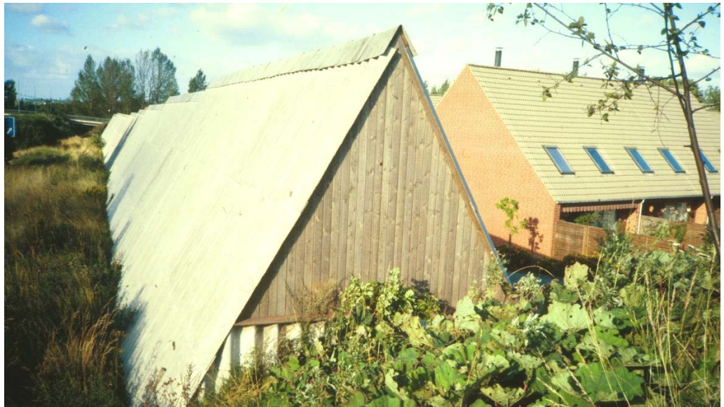
Figure 7.2. A new district of row houses constructed along an existing highway. A common carport facility was constructed as a two storey high noise barrier.
