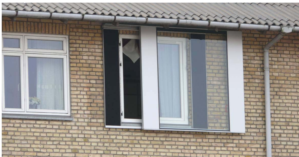
Figure 6.10. Close up of “noise shutter” window where the extra noise insulating glass layer can be pulled to the right side in order to be able to open the “original window” (photo Allan Jensen, Rambøll).
