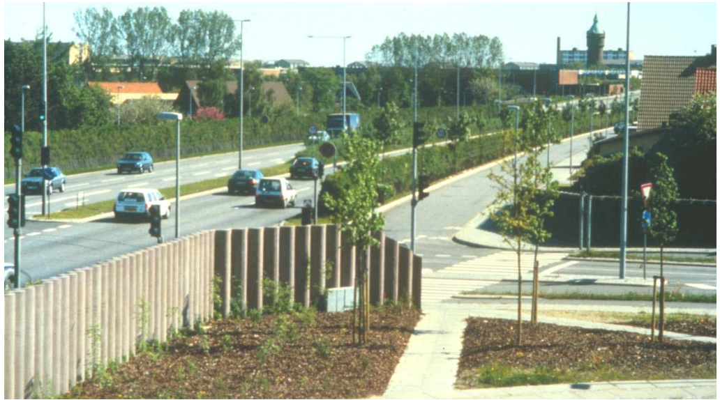
Figure 4.4. Combination of wave shaped concrete noise barrier and green noise barrier constructed as a "supported" earth wall along the new ring road in Århus, Denmark.
