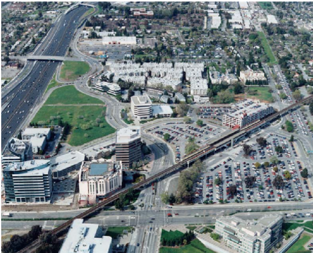
Figure 5.3. The Pleasant Hill BART District station and surroundings.
