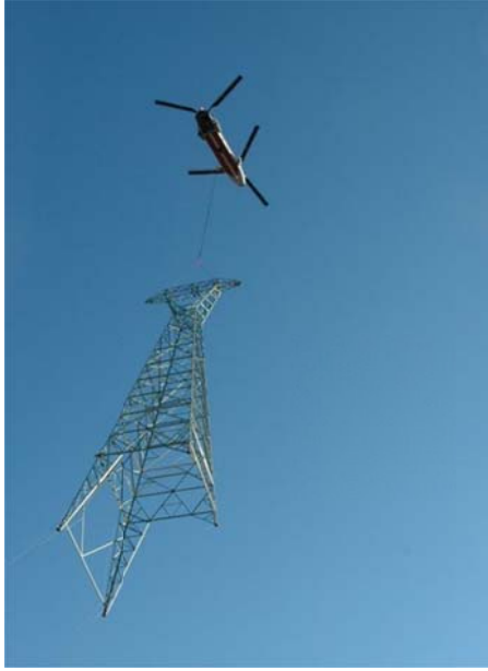
Figure 60: Boeing Chinook 234 helicopter lifting replacement asymmetrical tower.
