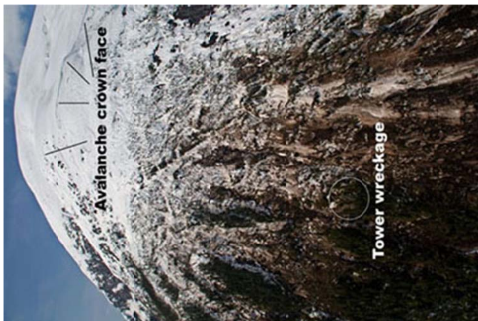
Figure 59: Photograph showing the crown face of the April 16, 2008 avalanche and location of Snettisham transmission line damage that it caused (KTOO, 2009).
