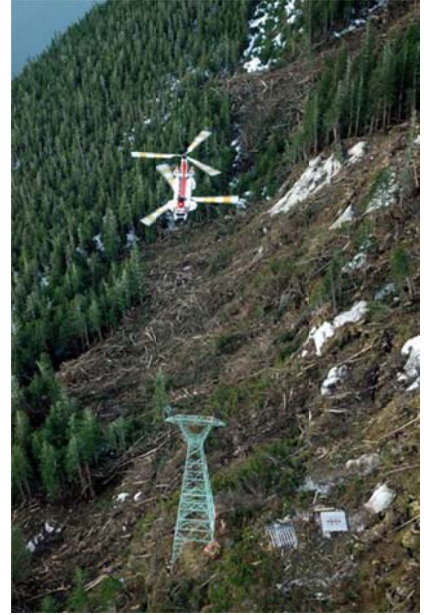
Figure 62: Boeing Chinook 234 helicopter sets replacement tower replacement onto intact original foundations.
