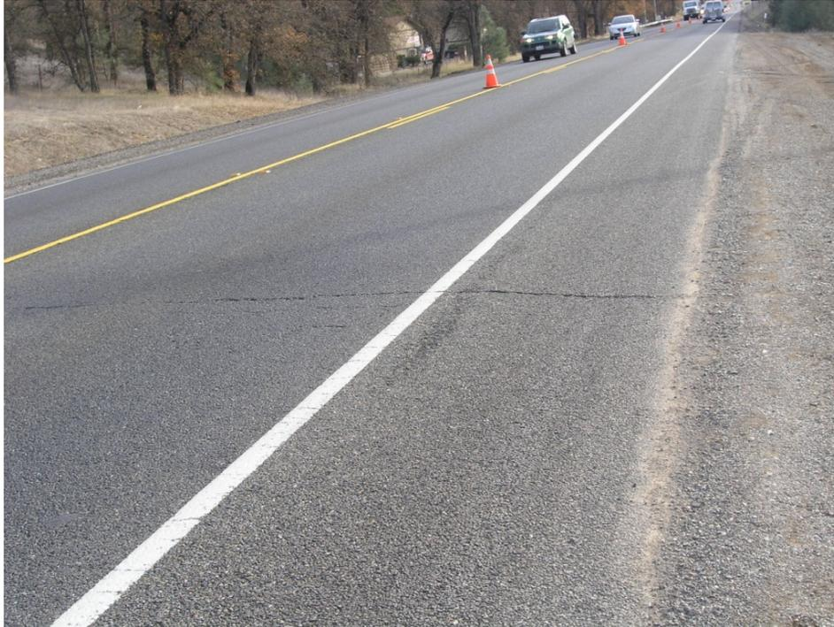
**Figure 7: Lake 53 transverse crack (near PM 5.25 NB).**
