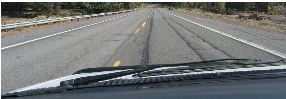
Figure 5: Two-lane section over causeway, approx. PM 10.4, EB.
