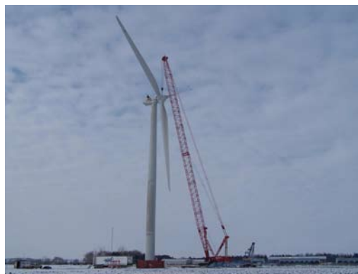
Construction of the 1.65 MW wind turbine at the Morris research center.
