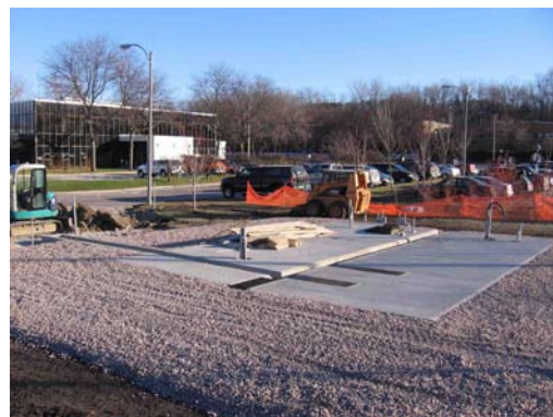
Demonstration site at the Vermont Department of Public Works in December 2005. This picture shows the platform ready for equipment to be installed.
