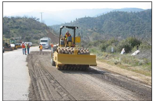
Figure 7.12: Padfoot impressions after multiple passes.
