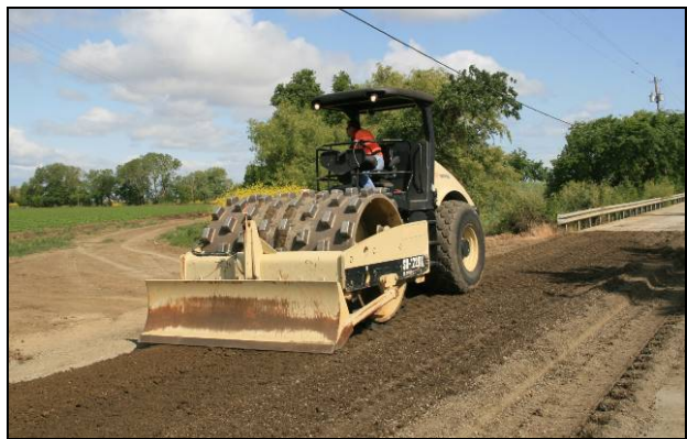
Figure 7.10: Using the blade to redistribute material in padfoot impressions.
