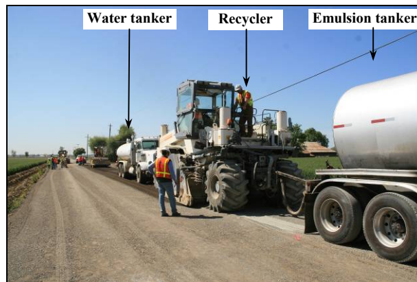
(c) Rotary mixer/recycler coupled to emulsion tanker and water tanker
