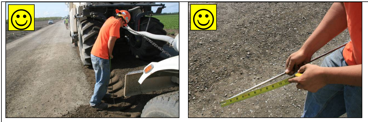
Figure 7.5: Checking mixing depth.
