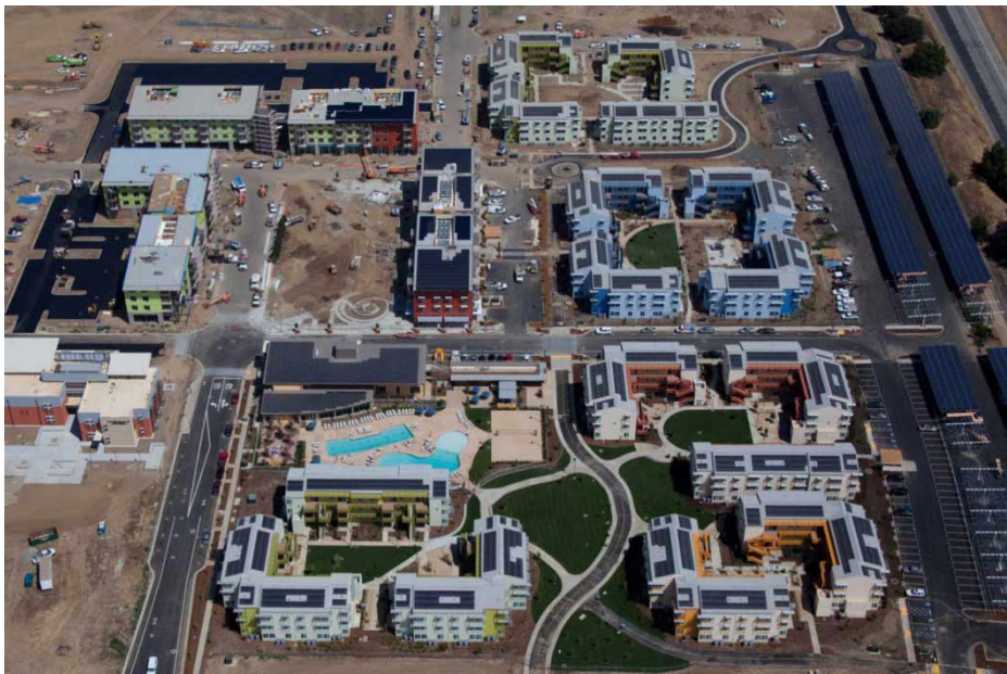
Figure 2. Aerial view of West Village under construction. West Village consists of 1,015 student housing units in three- and four-story apartment buildings and 475 faculty/staff housing units in townhouses and single family homes, grouped around a village square with commercial, social, recreational, and community college facilities. Source: Carmel Partners.
