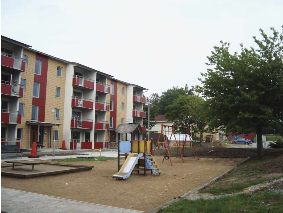
Figure 6. Public spaces. The community atmosphere is maintained throughout the renovations. Source: Carley Friesen.
