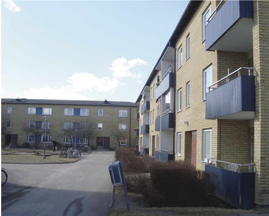
Figure 1. Apartments before. Successful courtyard typology; problems with thermal bridges from inset balconies. Source: Carley Friesen.
