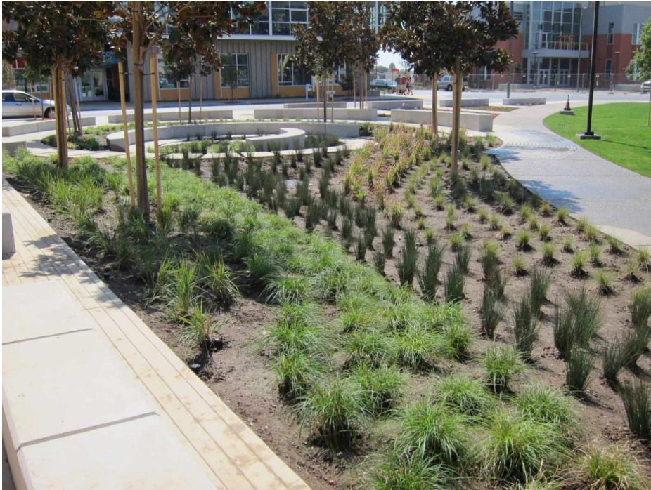
Figure 4. On-site drainage. Water from many public spaces at West Village drains first into swales planted with native vegetation, and then into a larger constructed wetland. Source: Photograph by Stephen M. Wheeler.
