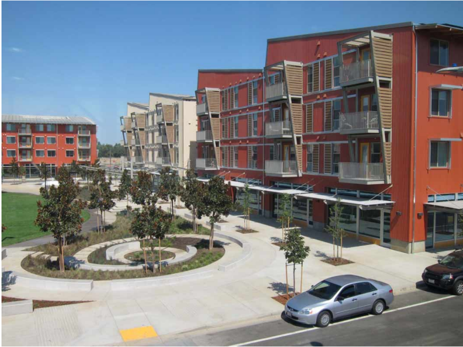
Figure 3. West Village Square. West Village is oriented around a central square. Building roofs are covered with photovoltaic panels, and strategically placed shades prevent the sun from overheating buildings. Source: Photograph by Stephen M. Wheeler.
