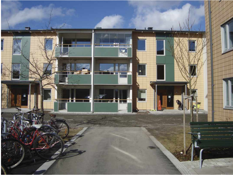
Figure 2. Apartments after. Maintained courtyard typology and look of facade while using new materials and fixing balconies. Source: Carley Friesen.
