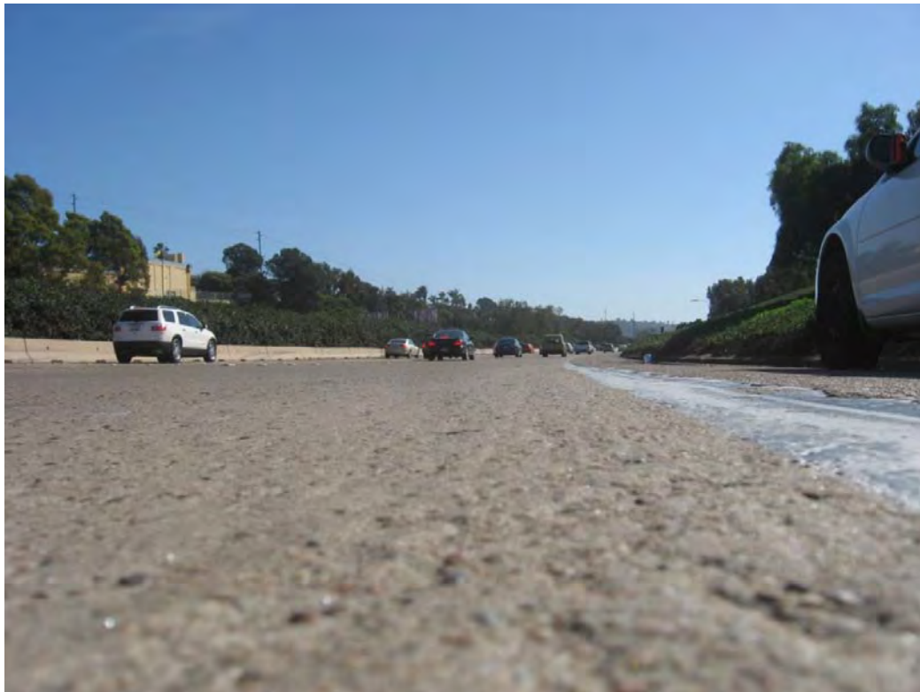
Figure A.2: Burlap drag, OBSI=107.3 dB(A) (Section QP-130.1).
