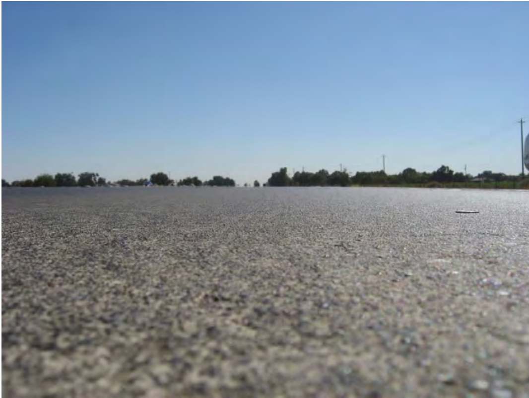
Figure A.1: Burlap drag, OBSI=103.0 dB(A) (Section QP-102.2).
