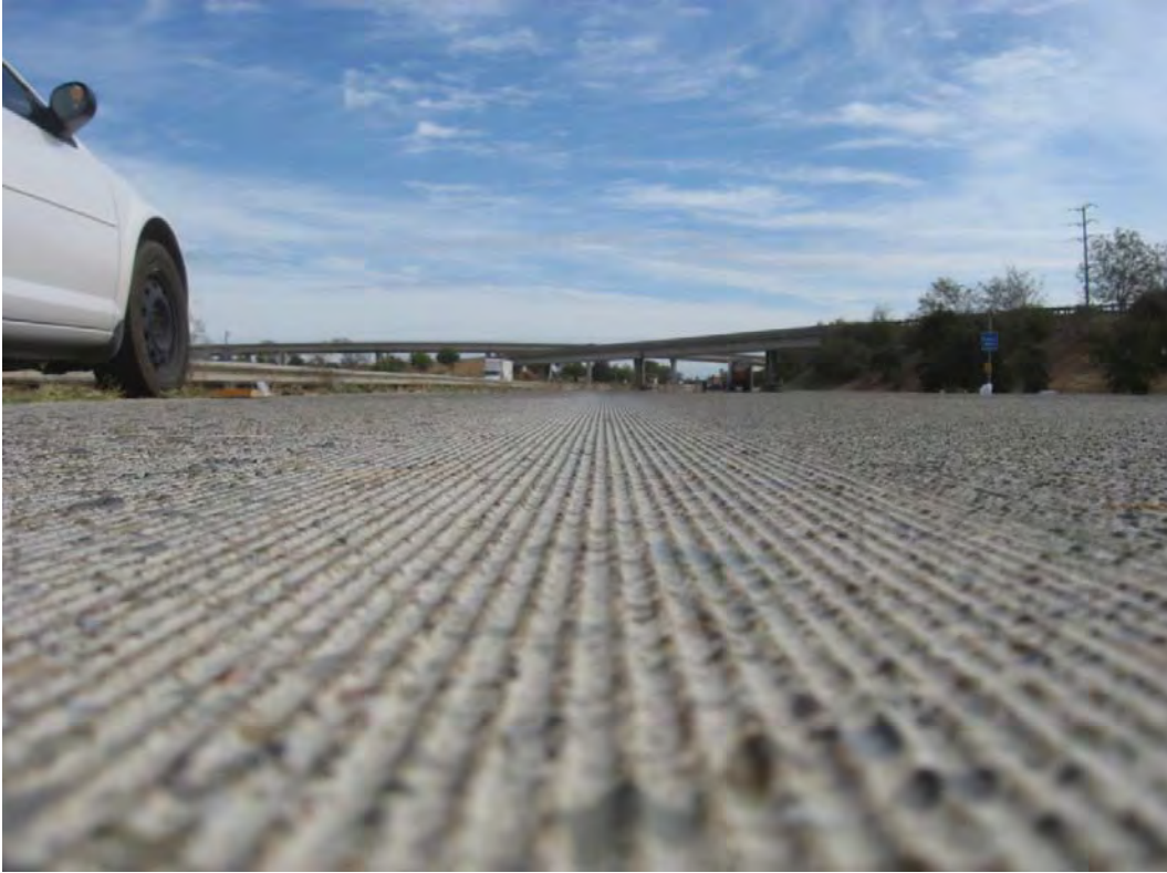
Figure A.3: Diamond ground, OBSI=99.4 dB(A) (Section QP-103.3).
