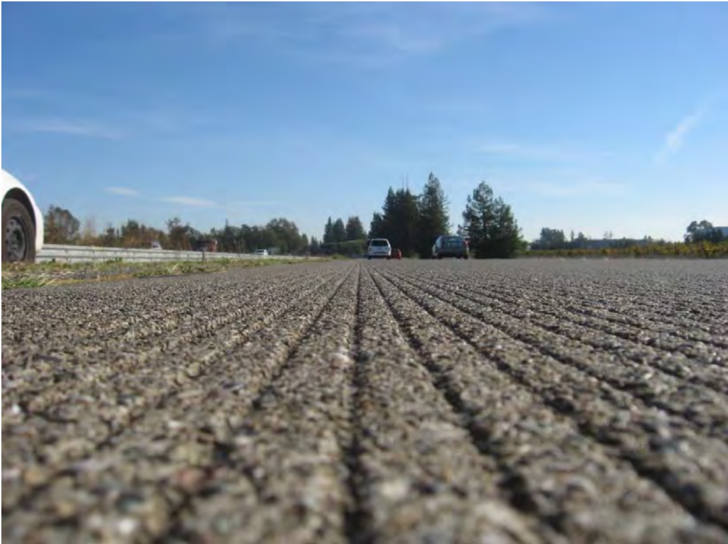
Figure A.5: Diamond grooved, OBSI=101.7 dB(A) (Section QP-138.3).
