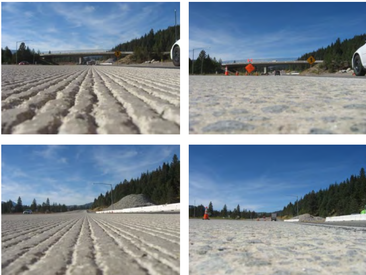
Figure C.1: Change in texture after one year at Sections QP-142.1 (top) and QP-142.3 (bottom).
