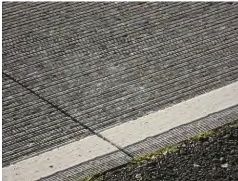
Texture and joint detail
