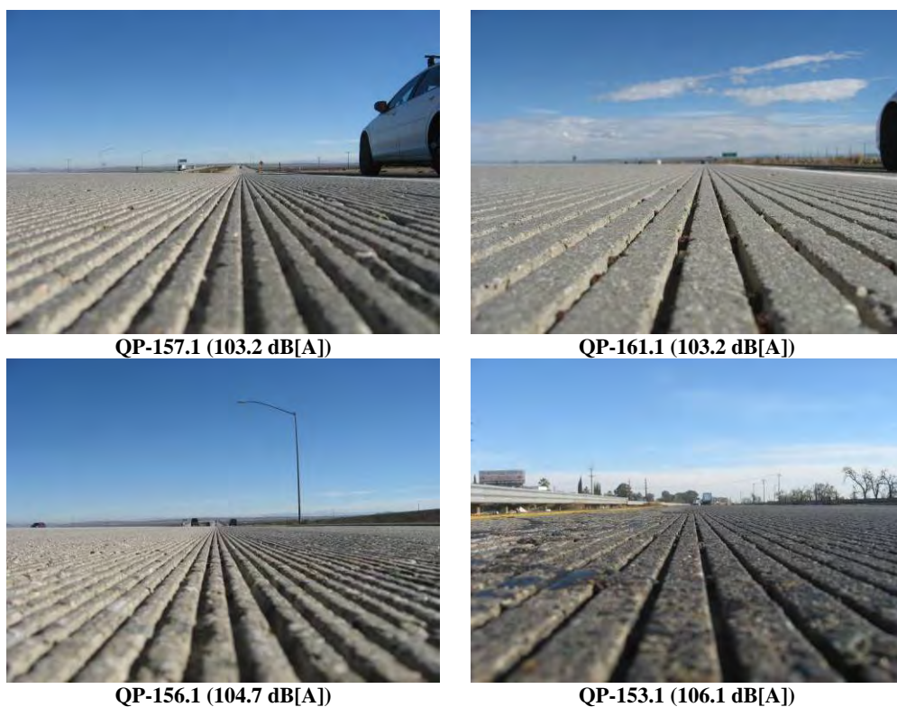
Figure 4.3: Example photographs of diamond grooved surfaces and their OBSI levels.
