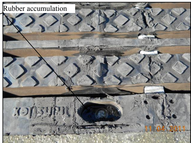
Figure 4.68: Phase 3.3: Tearing of rubber and accumulation of rubber particles in Trelleborg unit.
