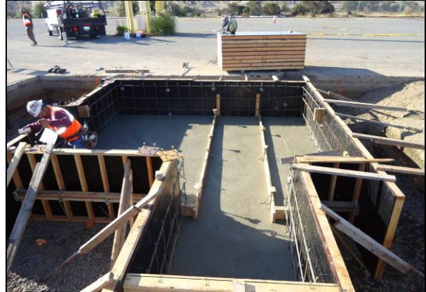
Figure 2.5: Formwork for test structure.
