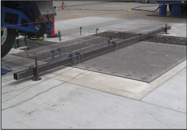
Figure 3.5: General view of instruments on top of structure.
