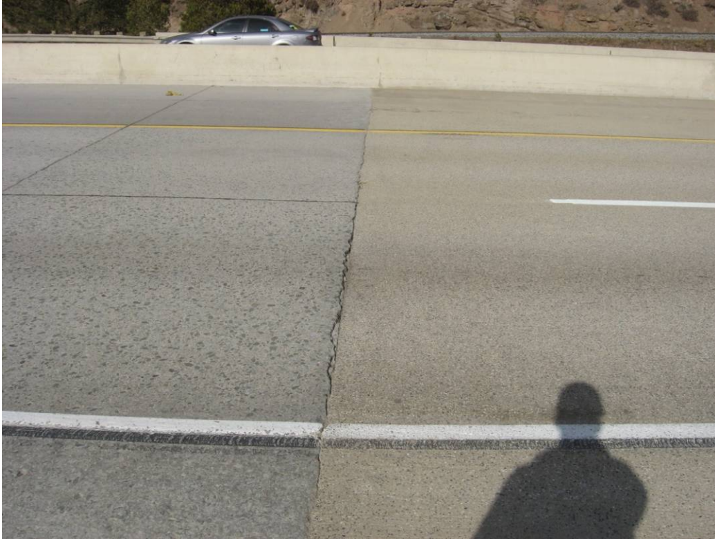
Figure 4.83: Beginning of Section QP-143.1 (right side of photo).
