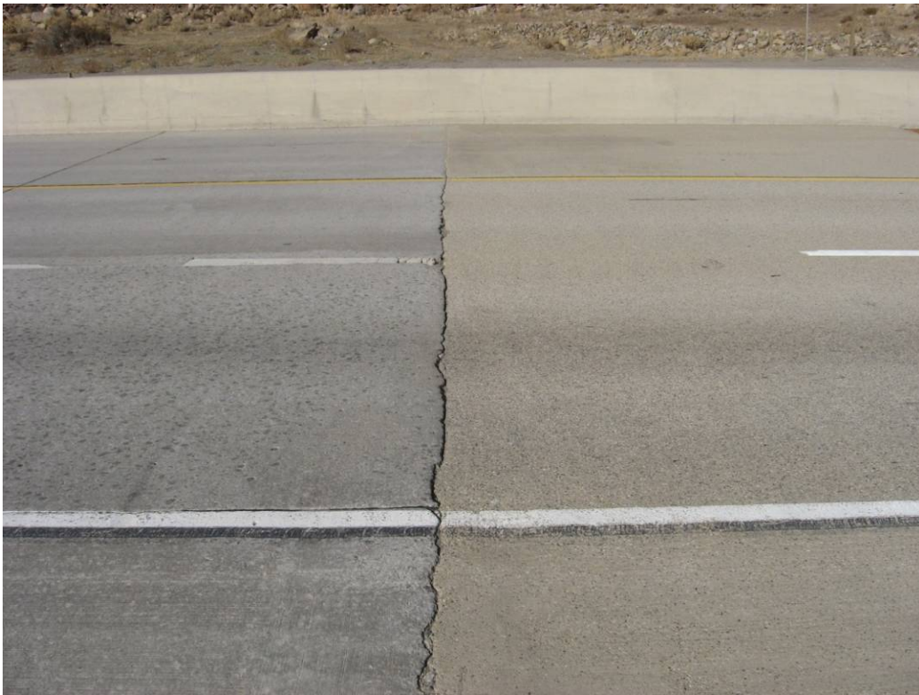
Figure 4.91: Pavement-bridge transition on Section QP-144.1 (right side of photo).
