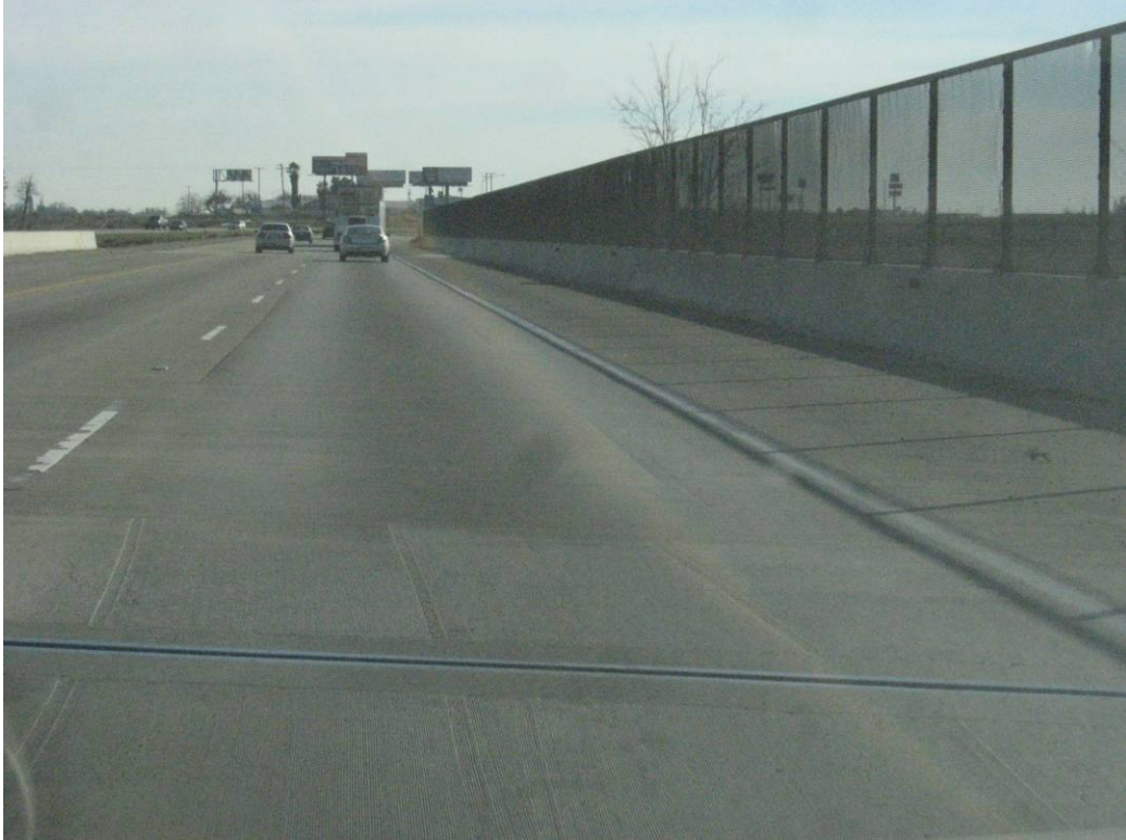
Figure 4.127: Beginning of Section QP-152.1 with diamond-ground surface near the joint.
