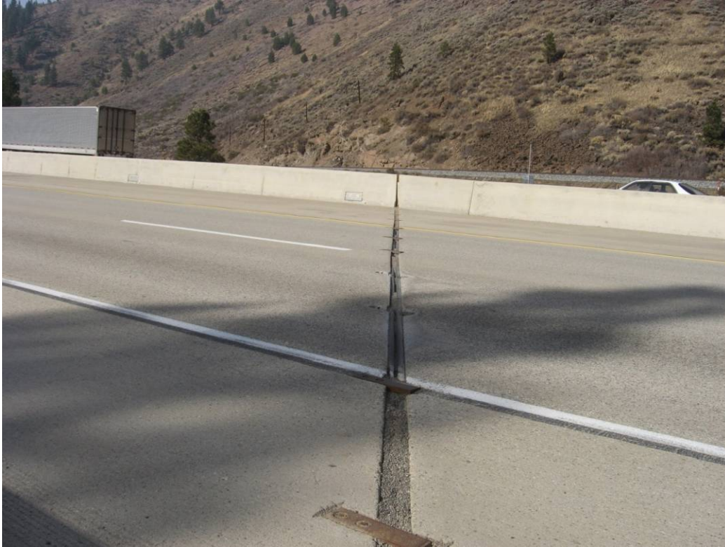
Figure 4.85: Joint on Section QP-143.1.
