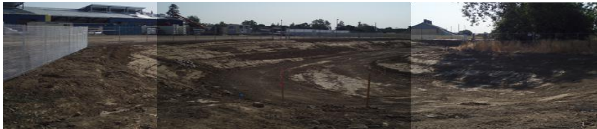
June 6, 2008- Southern drainage basin
