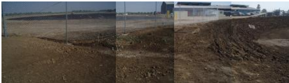
July 16, 2008- Southern drainage basin inlet
