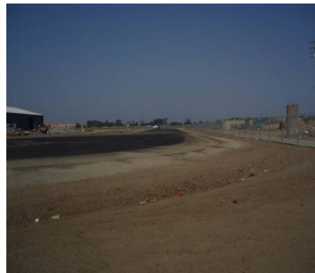
July 16, 2008- Northern edge, facing west; Shaping of road-side verge and swale
