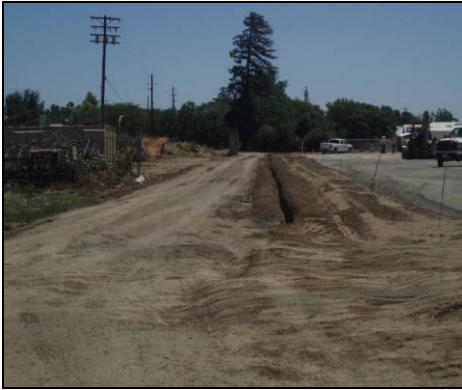
June 12, 2008: Northern edge, facing east- Gravel material added to track
