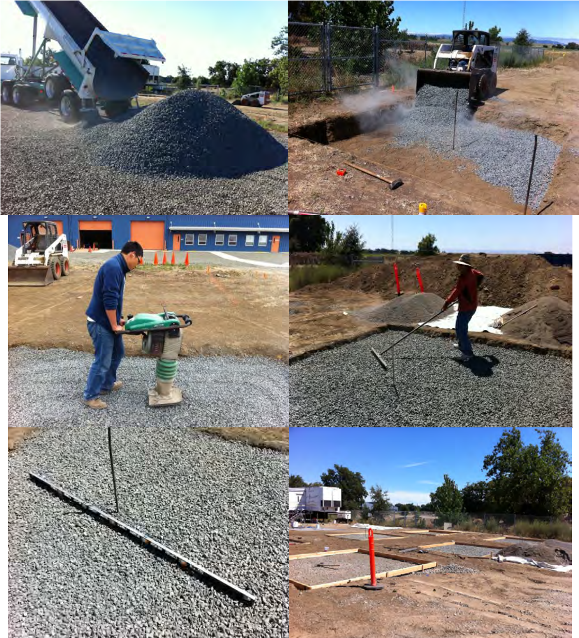
(b) Construction of base layers.
