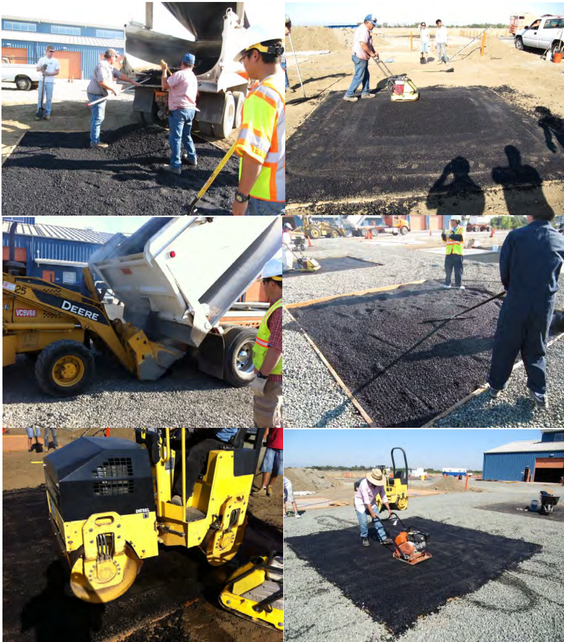
(e) Construction of surface layer (asphalt pavement).
