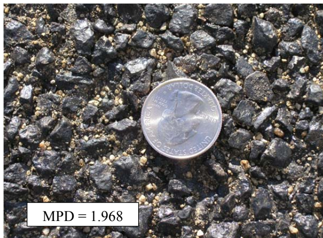
#2 Modified-binder seal coat - Modified gradation (PM 4.7-4.9)
