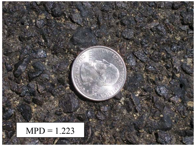
#6 1/4" PME seal coat - double chip seal (PM 10.0-9.8)
