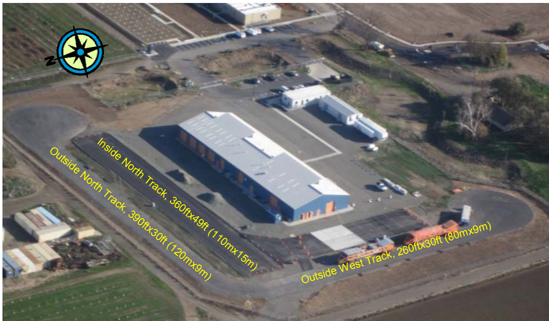
Figure 2.5: Aerial photo of the UC Davis ATIRC facility showing the test track locations and rough dimensions. The Outside North Track, Outside West Track, and a 360 ft long-by-16.4 ft wide area at the south part of Inside North Track were used for OGFC testing.
