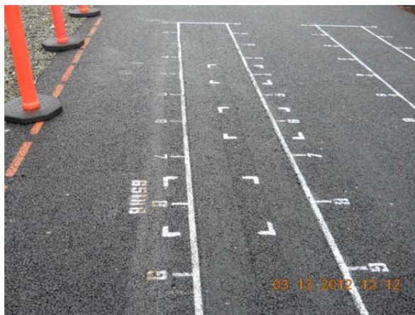
(a) 651HB: Georgia 1/2 inch mix with PG 58-34PM binder, OGFC thickness = 0.15 ft
