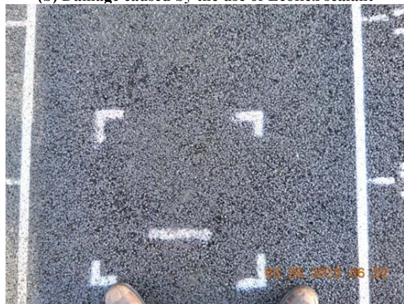
(d) Picture at Station 10 after HVS trafficking
