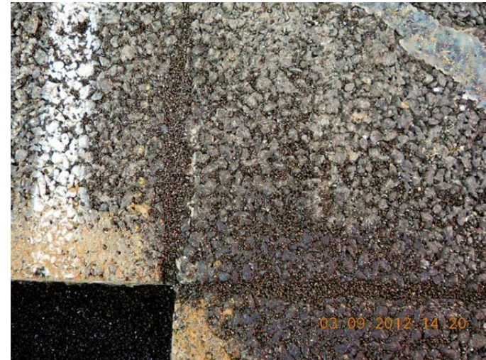
(e) Extended cuts in test sections refilled with emulsion-sand mixture
