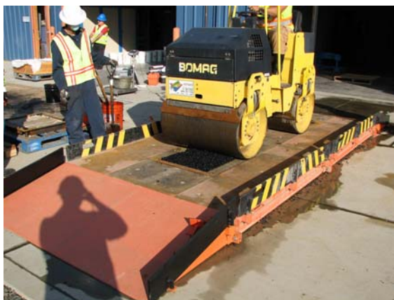
(a) Compaction using rolling wheel
