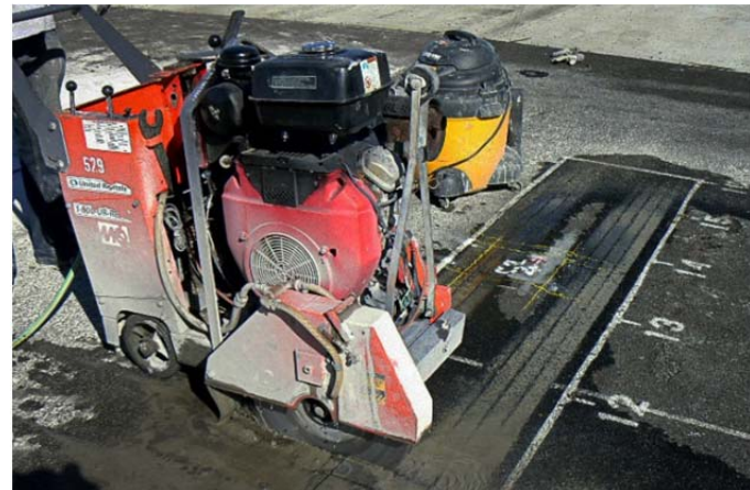
(i) Removal of scanned blocks for post-test scanning
