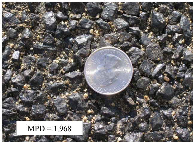
#2 Modified-binder seal coat — Modified gradation (PM 4.7-4.9)
