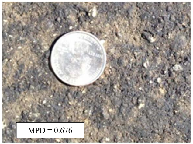
#8 Slurry seal (PM 9.4-9.6)
