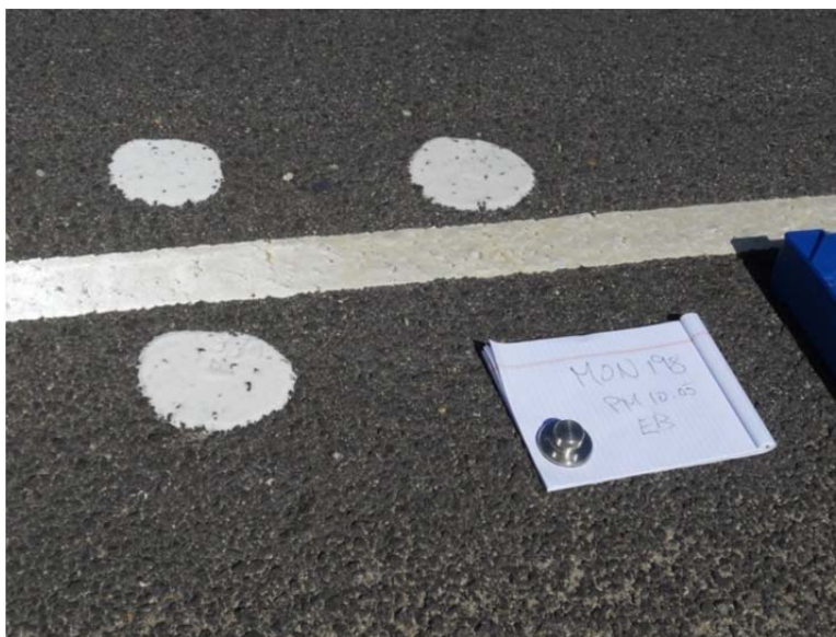
(b) Mon-198 PM 10.05 coarser 3/8" gradation chip seal
