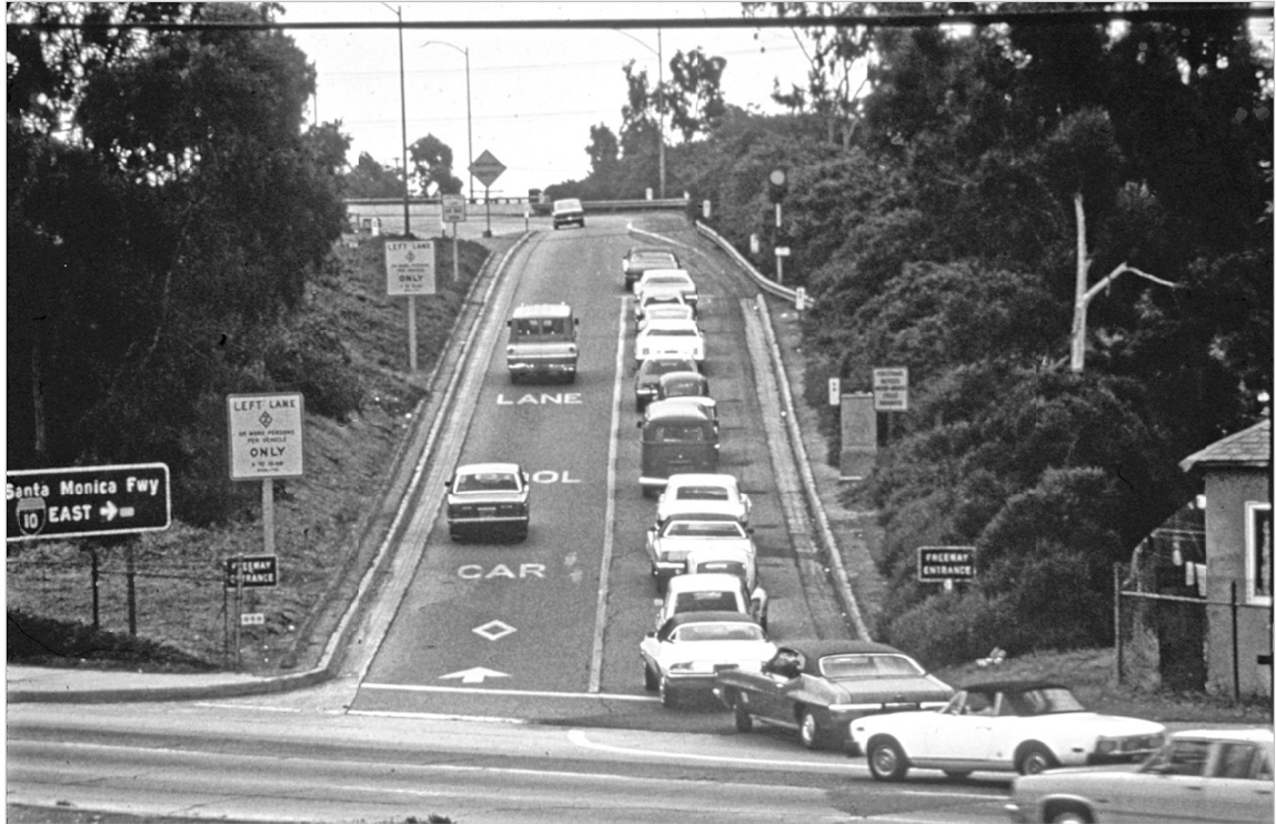
Figure 4 Single-occupancy vehicles queue at a ramp-metered entrance to Interstate 10 during the experimental diamond lane program.
