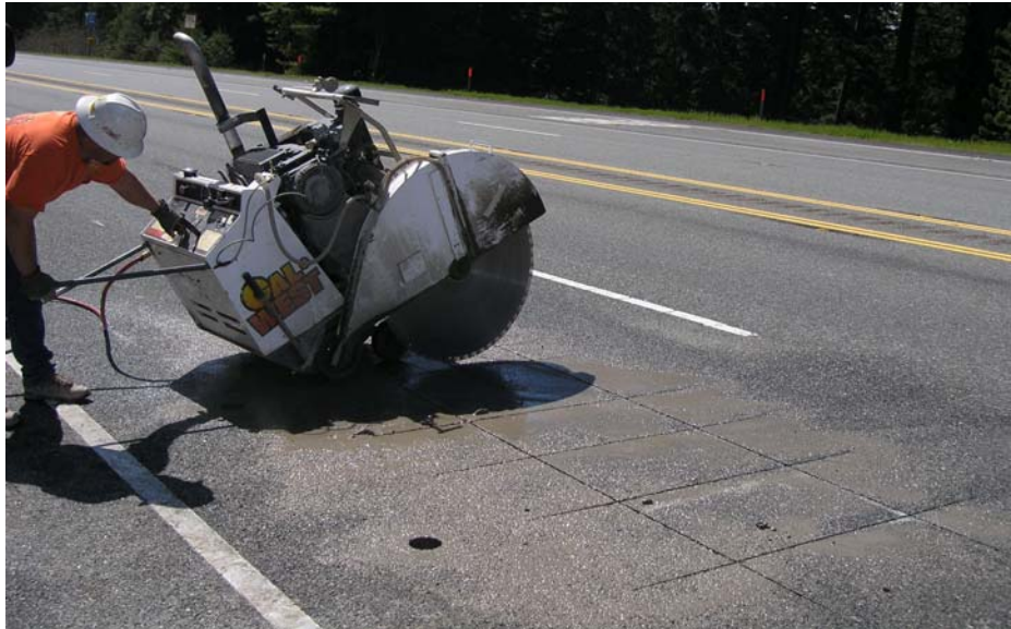
Figure 4.22: Cutting slabs of HMA layers from the pavement between wheelpaths.
