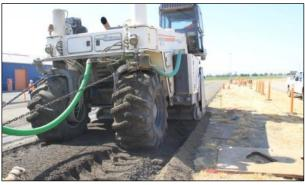
Figure 3.5: FDR-NS: Test track recycling.
