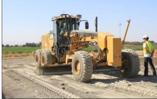
Figure 3.27: FDR-PC: Excess cement on Cell #7.
