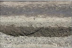
Figure 3.19: FDR-EE: Puddled water on surface after compaction.
