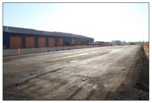
Figure 3.13: FDR-NS: Completed recycled layer surface.
