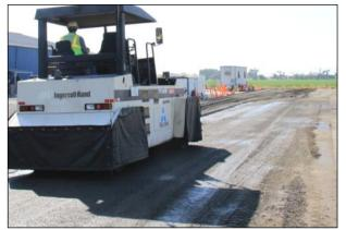
Figure 3.12: FDR-NS: Compaction with rubber-tired roller.
