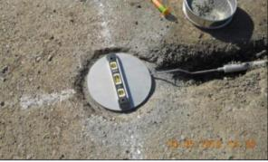
Figure 4.4: Pressure cell installation.
