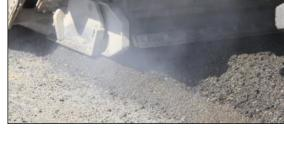
Figure 3.6: FDR-NS: Chunks at start of test pulverization.
