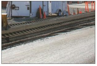
Figure 3.32: FDR-PC: Uniform mix after second recycling pass.
