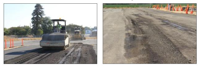
Figure 3.18: FDR-EE: Excess fluid during and after compaction with smooth drum roller.
