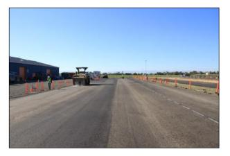
Figure 3.38: First lift of asphalt concrete after compaction.
