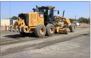
Figure 3.11: FDR-NS: Surface leveling with a grader.
