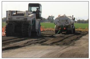
Figure 3.33: FDR-PC: Inconsistent mix on high cement content cells.
