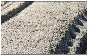
Figure 3.8: FDR-NS: Pulverized material.
