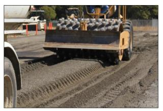
Figure 3.24: FDR-FA: Padfoot roller compaction on uniform mix.
