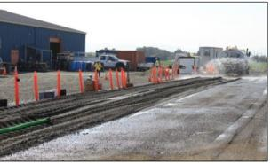
Figure 3.30: FDR-PC: Water spray prior to second mixing pass.
