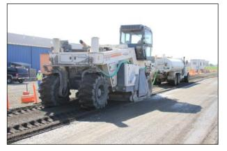
Figure 3.31: FDR-PC: Second mixing pass with water.
