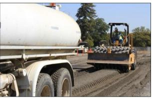
Figure 3.9: FDR-NS: Initial compaction with padfoot roller.
