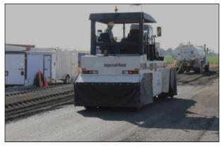
Figure 3.26: FDR-FA: Final compaction showing tightly bound surface.
