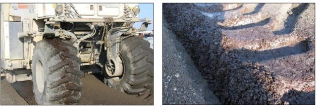
Figure 3.16: FDR-EE: Excess emulsion applied during recycling.
