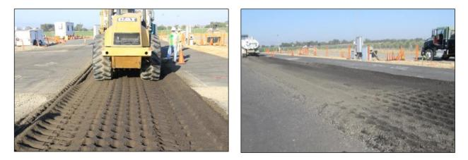
Figure 3.17: FDR-EE: Compaction with padfoot roller. (Note untreated areas and emulsion adhering to tire).
