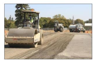
Figure 3.10: FDR-NS: Compaction with smooth drum roller.
