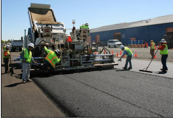
Figure 2.37: Cecabase: No smoke from truck and paver.
