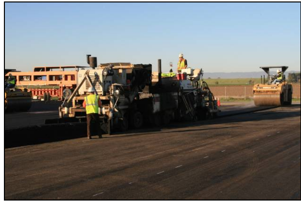
Paving and breakdown rolling
