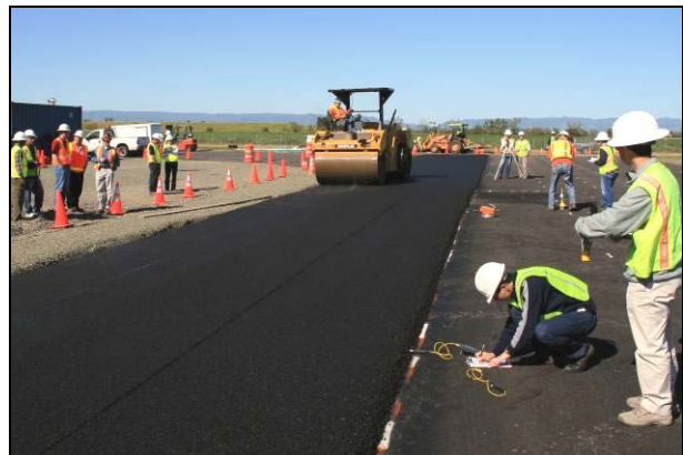
Figure 2.33: Gencor: Breakdown rolling.
