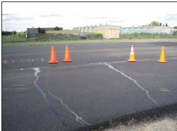
Figure 2.48: Water seepage from Cecabase section.
