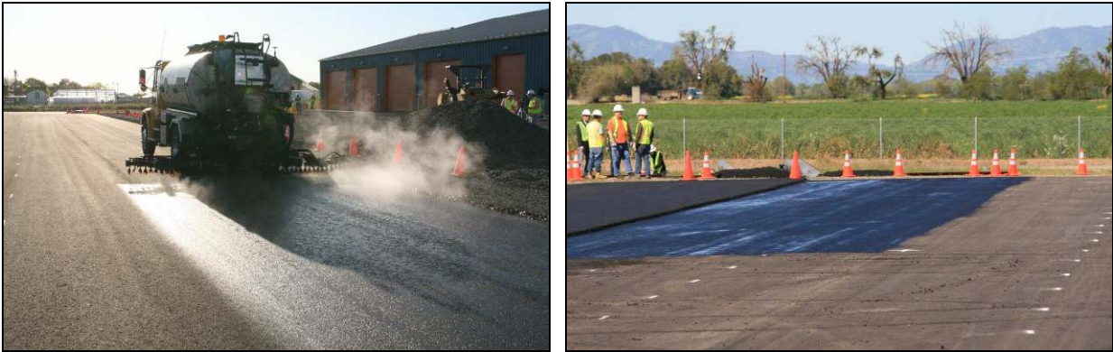
Figure 2.27: Tack coat application.
