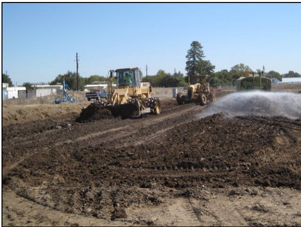
Figure 2.8: Watering and mixing.
