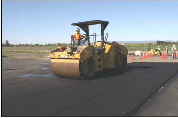
Figure 2.30: Control: Breakdown rolling.
