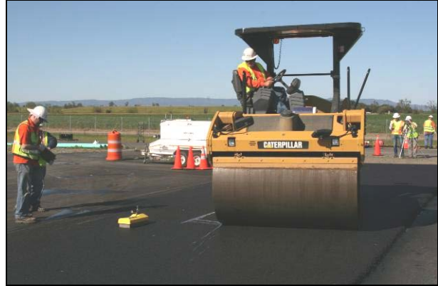
Figure 2.31: Control: Final rolling.
