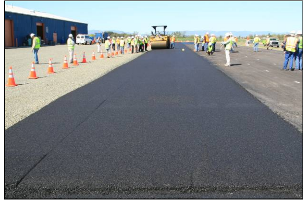
Figure 2.35: Evotherm: Breakdown rolling.
