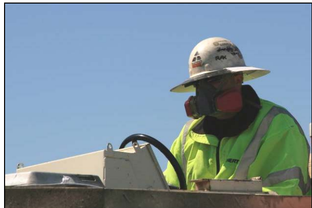
Figure 2.29: Control: Paver operator wearing respirator.
