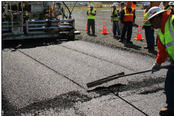
Figure 2.36: Evotherm: Improved workability.
