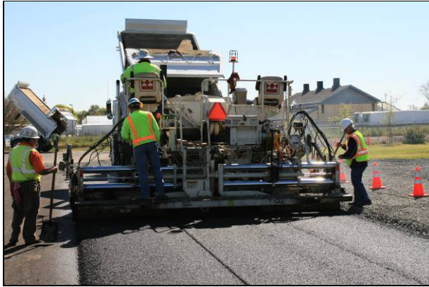
Figure 2.34: Evotherm: No smoke from truck and paver.
