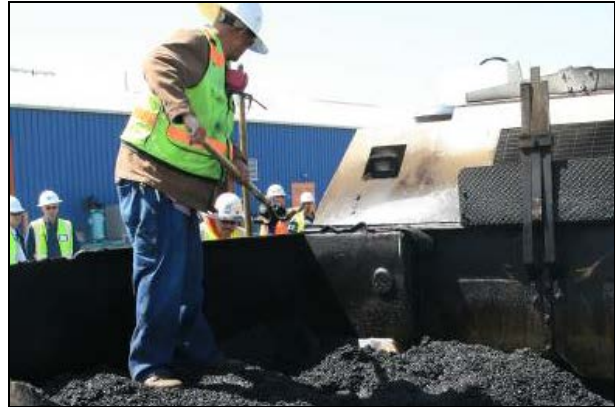
Figure 2.36: Advera: Removing chunks from paver.
