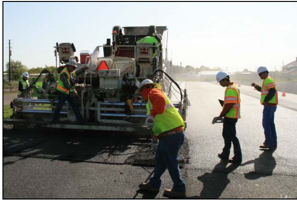
Figure 2.41: Astec: Some smoke from truck and paver.
