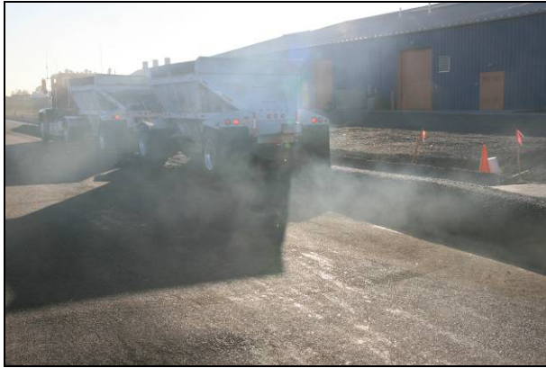
Placing asphalt in windrow
