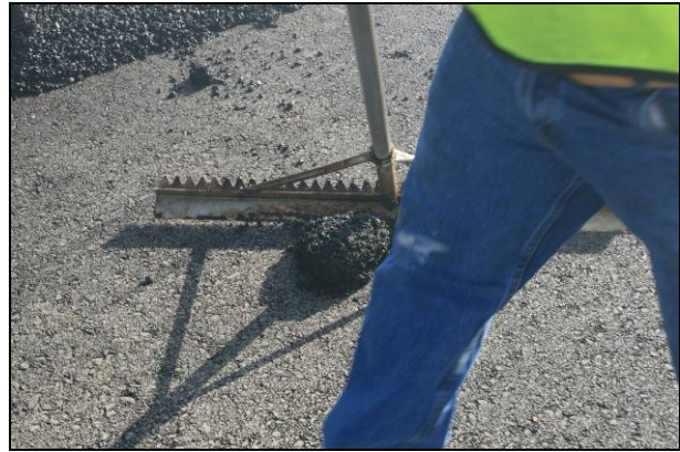
Figure 2.39: Control #2: Chunks removed from section.
