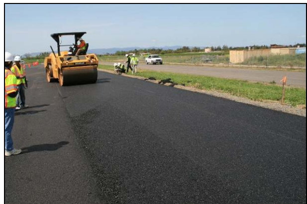
Figure 2.44: Rediset: Breakdown rolling.
