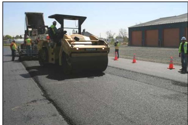
Figure 2.34: Sasobit: Breakdown rolling.
