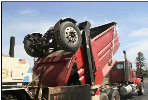
Figure 2.43: Rediset: No smoke from truck or paver.
