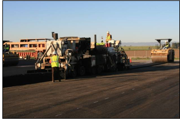
Paving and breakdown rolling
