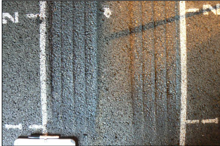
Figure 4.20: 625HA: Section photograph at test completion.
