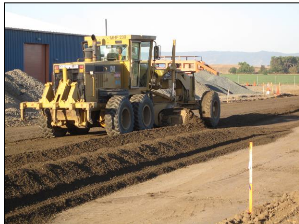
Figure 2.16: Material spreading.
