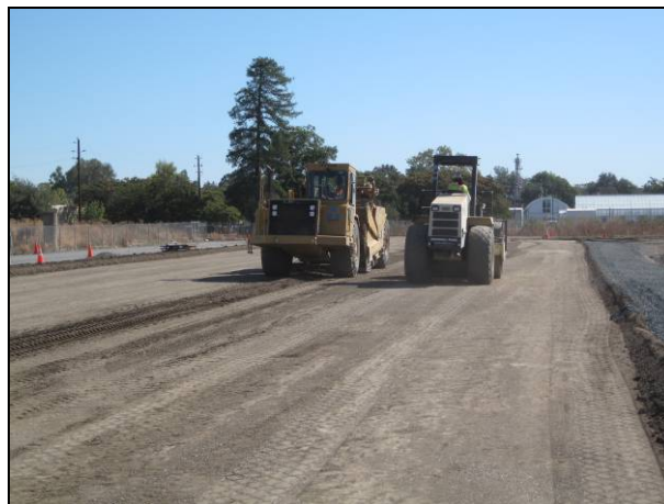
Figure 2.19: Heavy watering prior to pre-final compaction.
