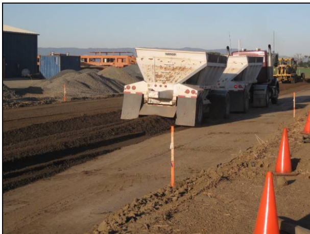
Figure 2.15: Dumping material in windrows.
