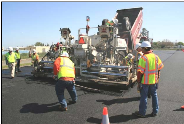
Figure 2.33: Sasobit: Absence of smoke from truck and paver.
