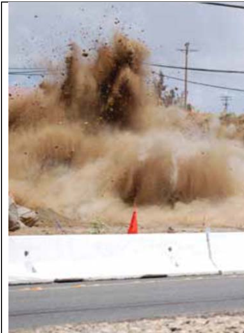
Figure 18. Bedrock blasting for SR-76 Middle (2010)
