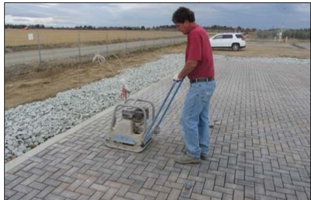
Figure 5.15: Paver placement and compaction.
