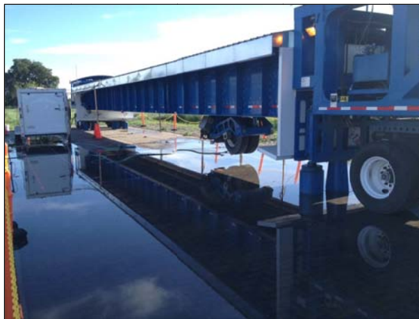
Figure 6.14: Flooded section during preparation for wet testing.
