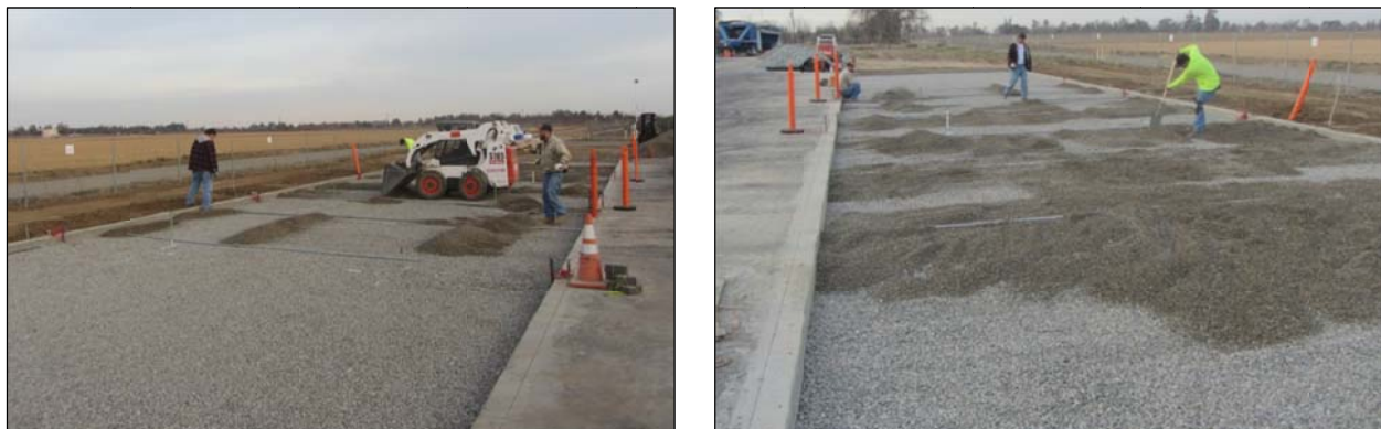
Figure 5.14: Bedding layer placement.
