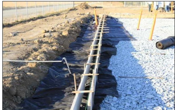
Figure 5.9: Formwork for curb.
