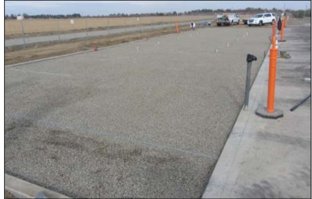
Figure 5.13: Bedding layer placement.
