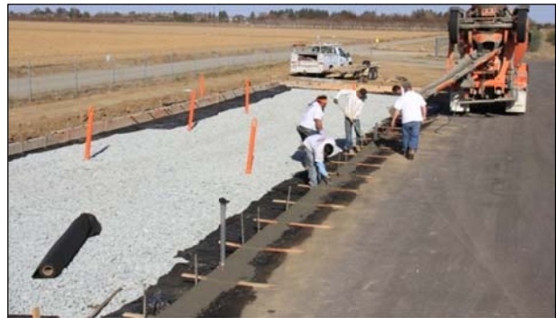
Figure 5.9: Formwork for curb.
