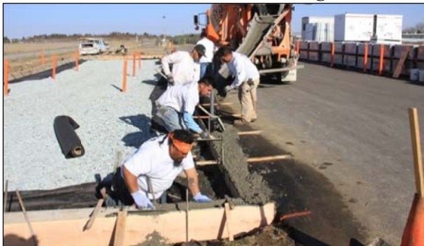
Figure 5.9: Formwork for curb.
