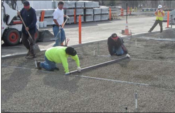
Figure 5.13: Bedding layer placement.
