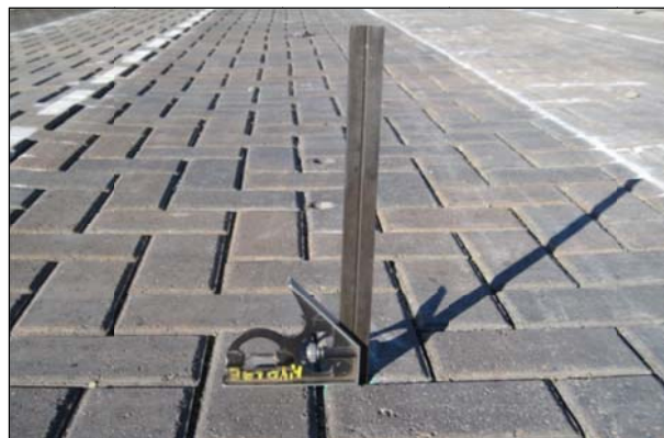
Figure 6.13: Jointing stone depth measurement.
