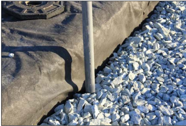
Figure 6.3: Perforated pipe for water level measurements.
