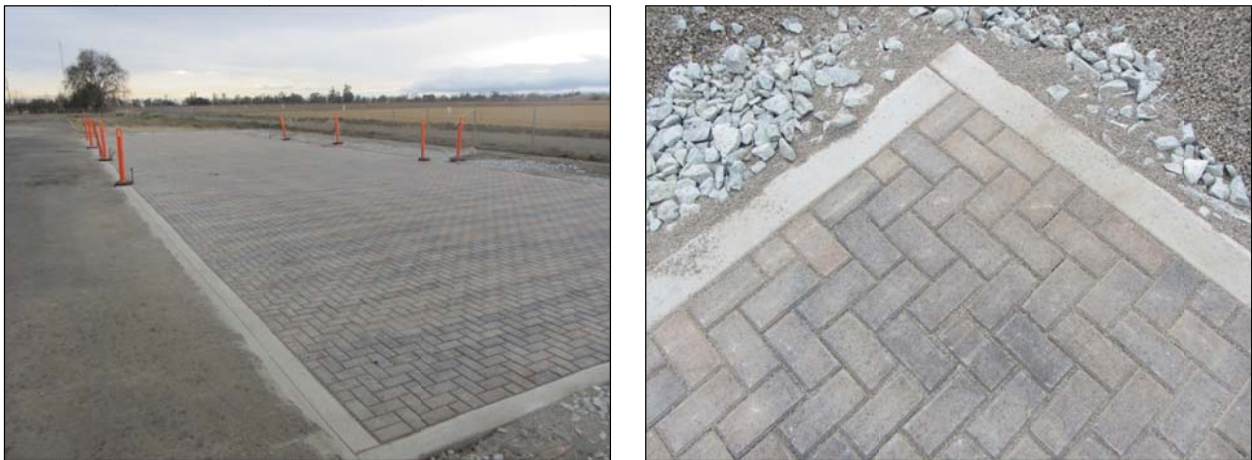
Figure 5.17: Completed test track.
