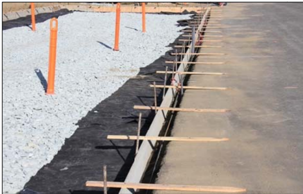
Figure 5.9: Formwork for curb.
