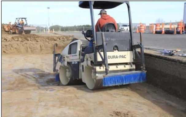
Figure 5.2: Subgrade compaction.
