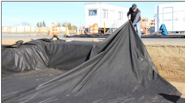
Figure 5.7: Geotextile placement.
