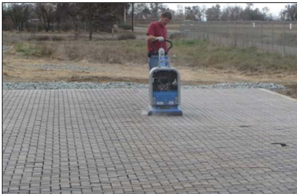
Figure 5.15: Paver placement and compaction.
