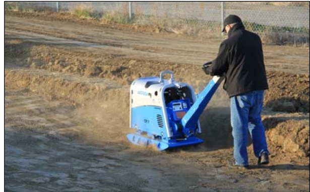
Figure 5.2: Subgrade compaction.
