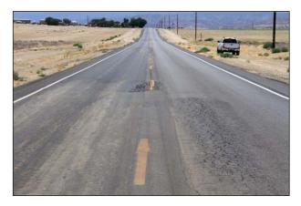
Figure 2.5: Fatigue cracking.
