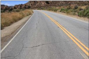
Figure 2.3: Block cracking.
