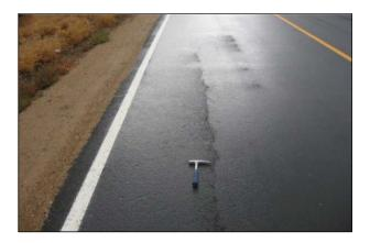
Figure 2.2: Longitudinal crack.
