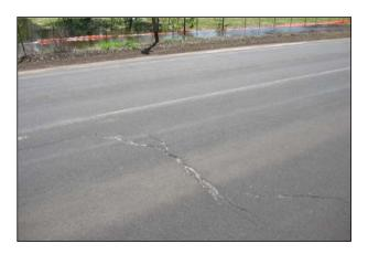
Figure 2.1: Transverse crack.
