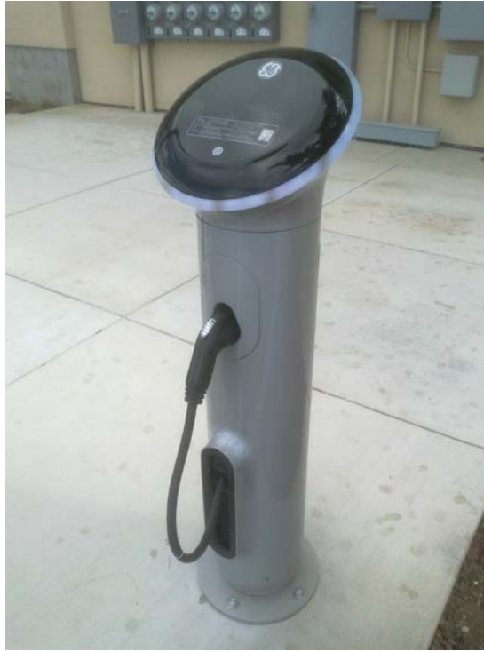
Figure 15: Electric Vehicle Charging Post
