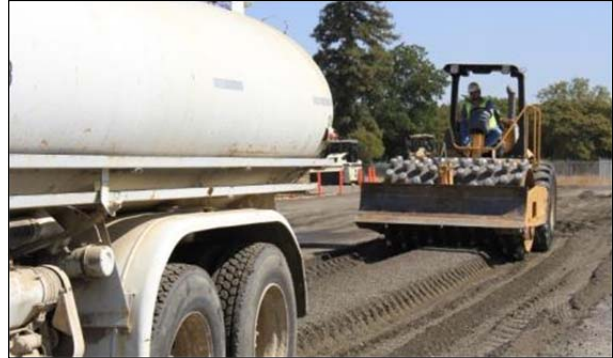
Figure 3.9: FDR-NS: Initial compaction with padfoot roller.
