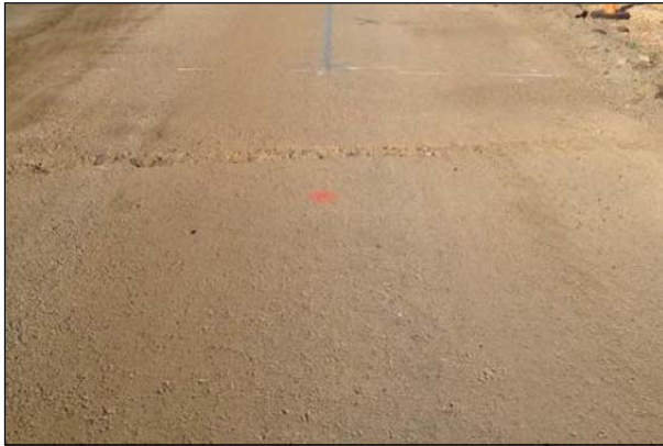
Figure 3.34: Broomed surface of FDR-NS layer.
