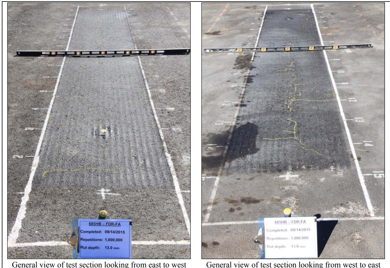
Figure 6.14: 685HB: Test section photographs.
