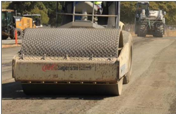
Figure 3.25: FDR-FA: Steel wheel compaction showing tightly bound surface.
