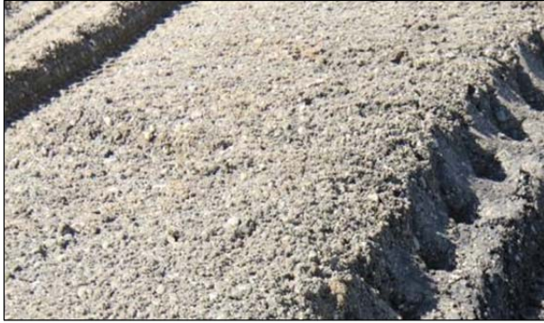
Figure 3.8: FDR-NS: Pulverized material.
