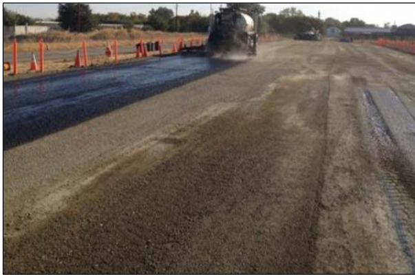
Figure 3.34: Broomed surface of FDR-NS layer.
