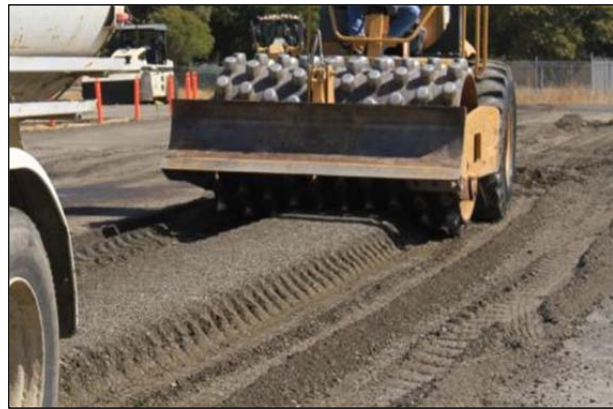
Figure 3.24: FDR-FA: Padfoot roller compaction on uniform mix.
