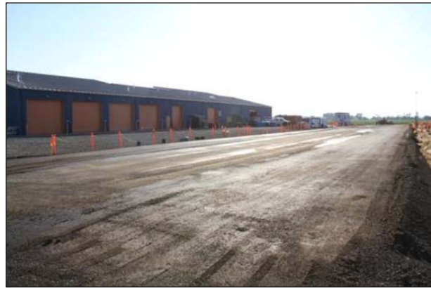
Figure 3.11: FDR-NS: Surface leveling with a grader.
