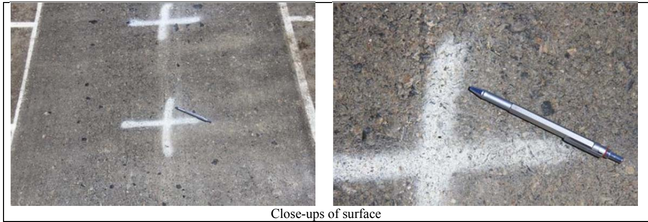
Figure 5.64: 674HB: Test section photographs.
