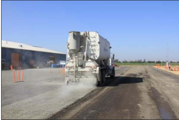
Figure 3.21: FDR-FA: Spreading cement on old asphalt surface.
