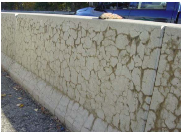
Figure A.2: Example photos showing some of the common petrographic features of ASR.
