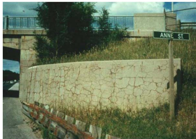
Figure A.2: Example photos showing some of the common petrographic features of ASR.
