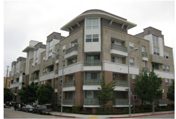
Photo by Texas A&M Transportation Institute
