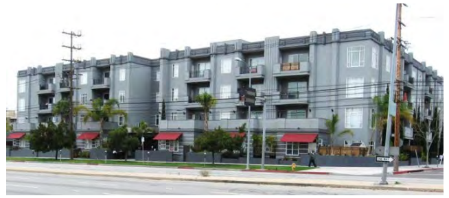
Photo by Texas A&M Transportation Institute
