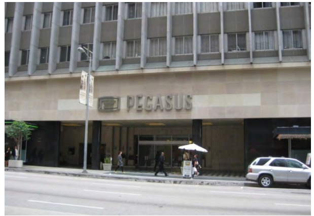
Photo by Texas A&M Transportation Institute
