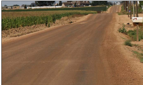
Figure 2.8: Road treated with petroleum resin.
