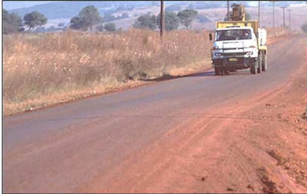
Figure 2.3: Road treated with calcium chloride.
