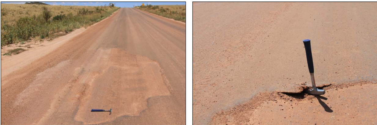
Figure 5.4: Effect of biscuit layer on treated surface.
