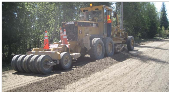
Figure 5.6: Grader-mounted roller.
