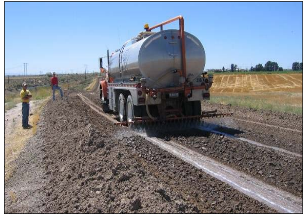
Figure 5.19: Spraying the chemical treatment.
