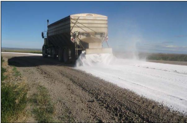
Figure 5.14: Flake application of calcium chloride.
