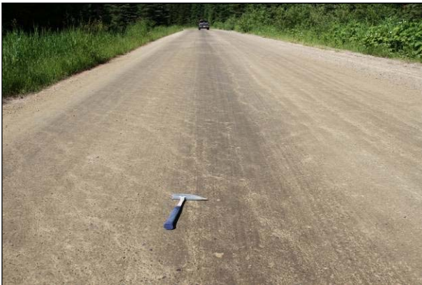
Figure 1.4: Treatment used to keep a good road in good condition.
