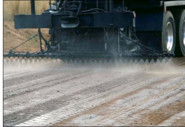
Figure 5.23: Light application of treatment to seal the surface.
