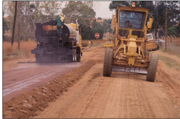
Figure 5.25: Blade mixing application.
