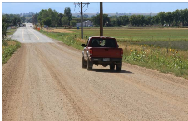
Figure 2.5: Road treated with glycerin-based product.
