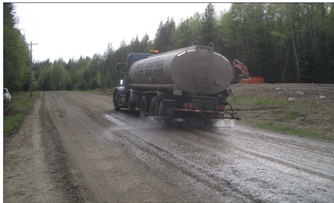
Figure 5.1: Applying a chemical treatment to a well-prepared road.
