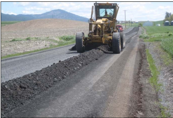
Figure 5.20: Shaping the road.
