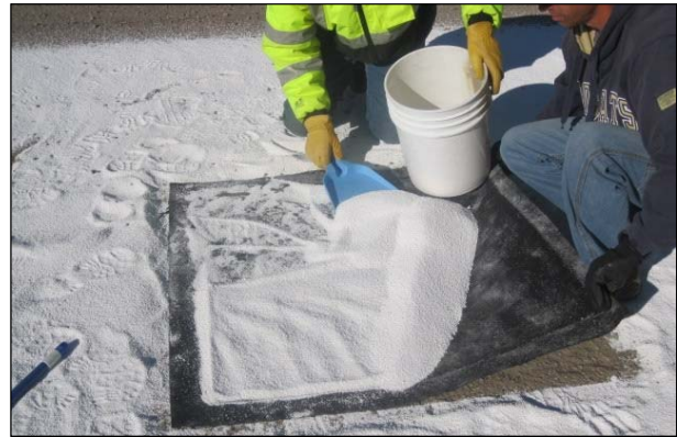
Figure 5.15: Checking application rate of calcium chloride flakes.
