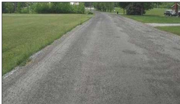
Figure 2.9: Road treated with synthetic fluid.
