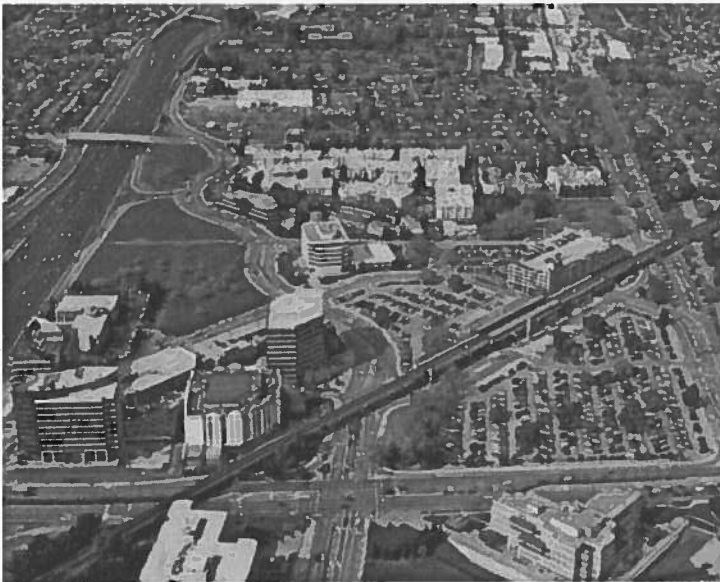
FIGURE 3: Pleasant Hill BART Station and Surroundings
