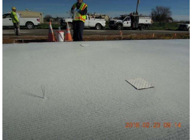
Appearance of the final surface
