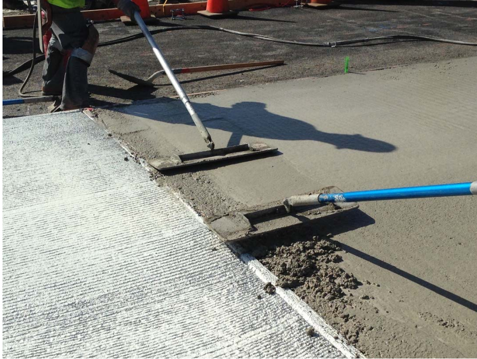
Figure A.59: Edge finishing.
