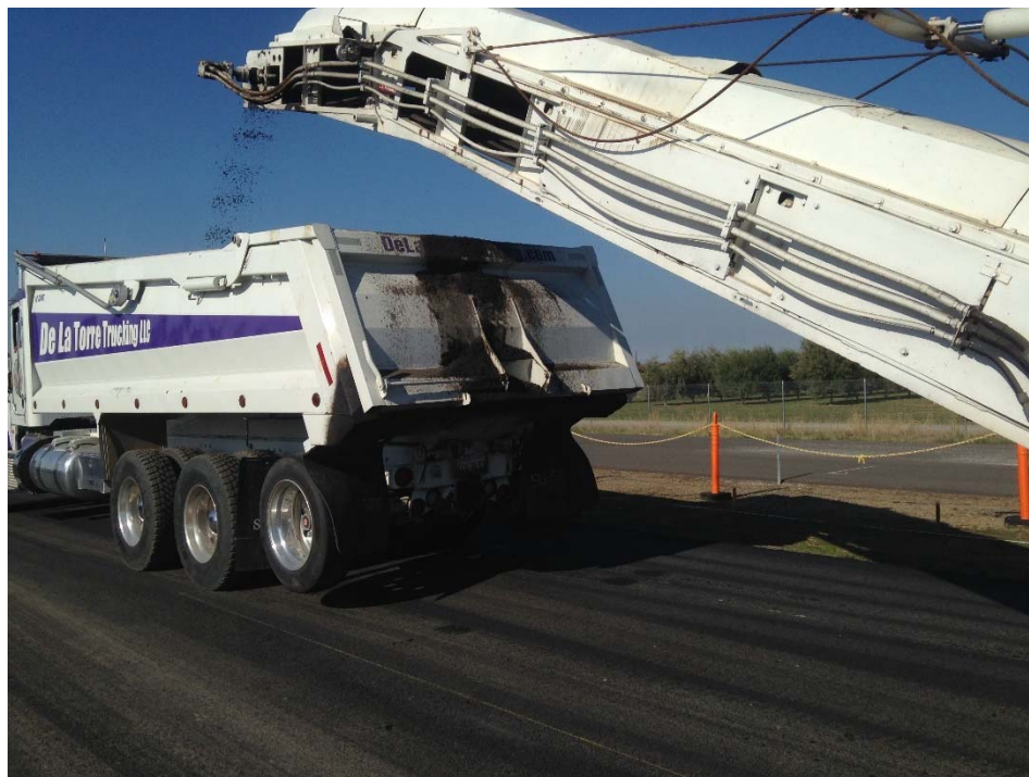
Figure A.10: Disposal of milled material.
