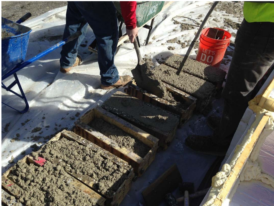
Figure A.60: Flexural beam preparation.
