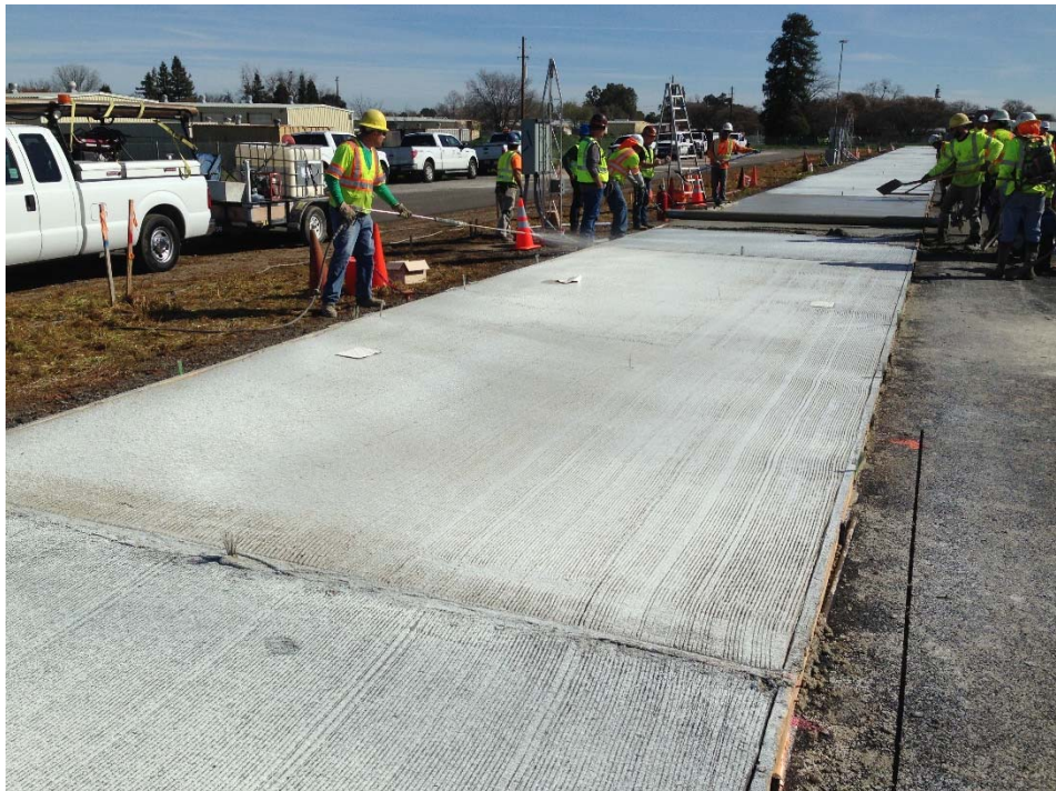
Figure A.72: Manual application of curing compound.
