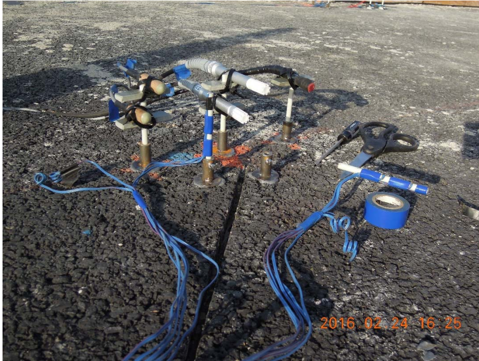
Figure A.29: From left to right: two moisture content sensors, thermocouples attached to a fiberglass rod, two RHC relative humidity sensors, and one RHS relative humidity sensor.
