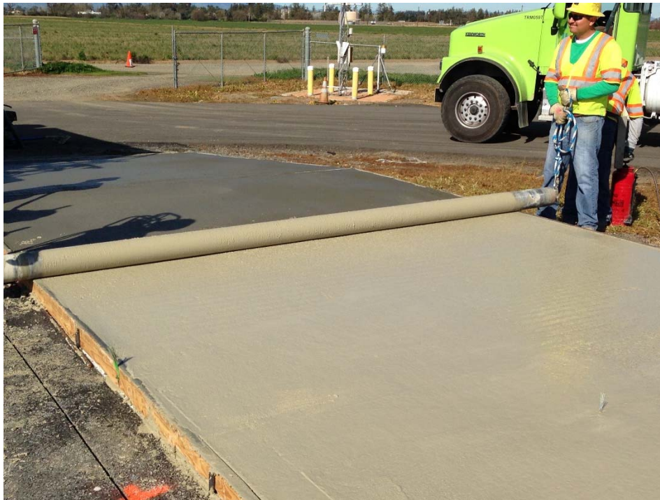
Figure A.55: CSA section after concrete consolidation.
