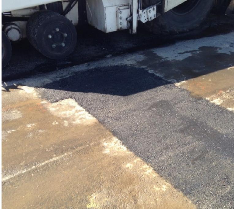
Figure A.7: Patch on distressed area of the test track.
