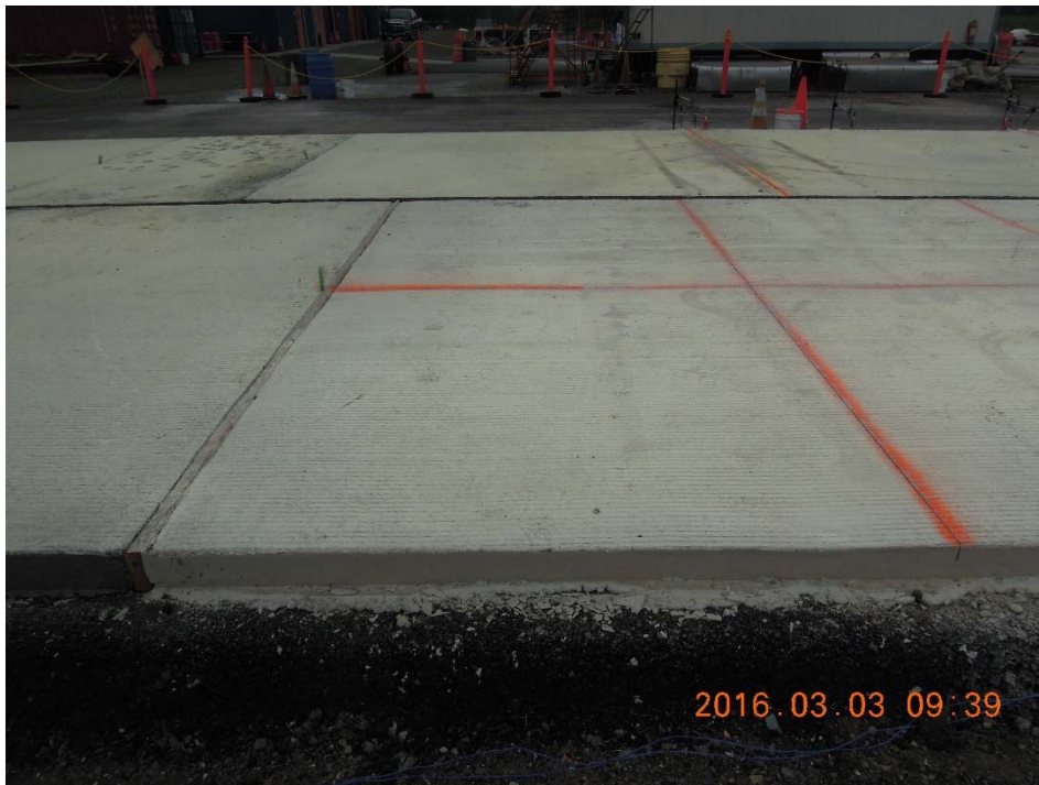
Figure A.102: Side view of Section H.
