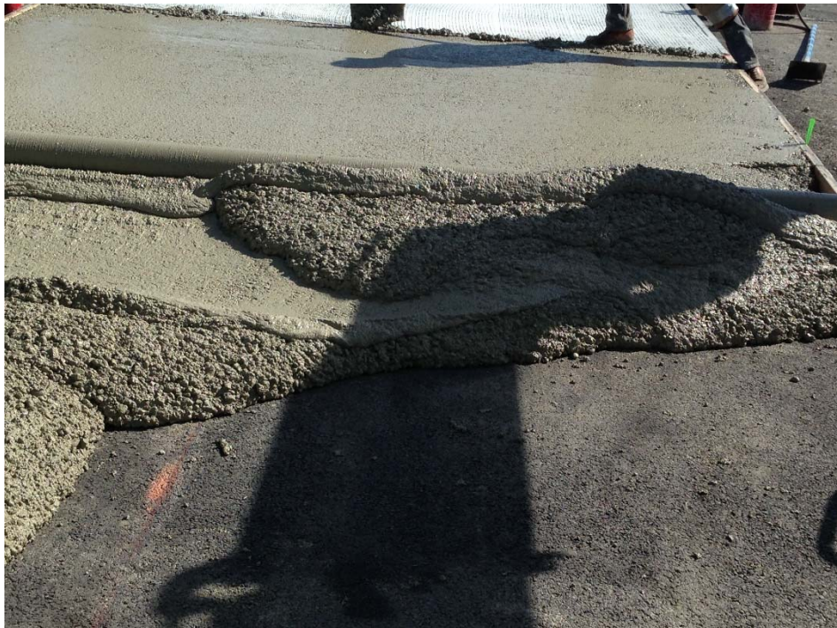
Figure A.58: P2 (Type II/V cement) concrete consolidation.
