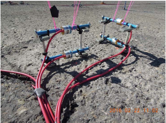
Static strain gages (two longitudinal, two transverse) Note: the pink threads will mark the exact location of the VWSGs after overlay paving. The exact location of the gages was required for forensic coring.
