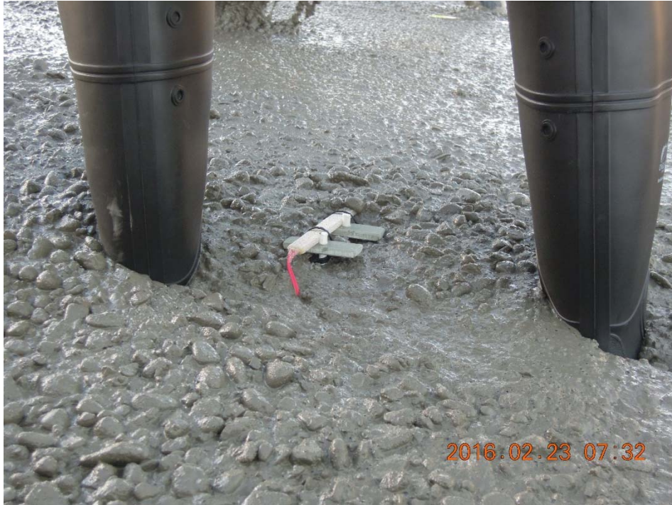
Figure A.37: Protecting the dynamic strain gages.
