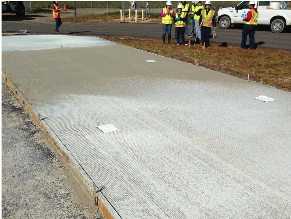
Figure A.64: Pads to measure the curing compound application rate.
