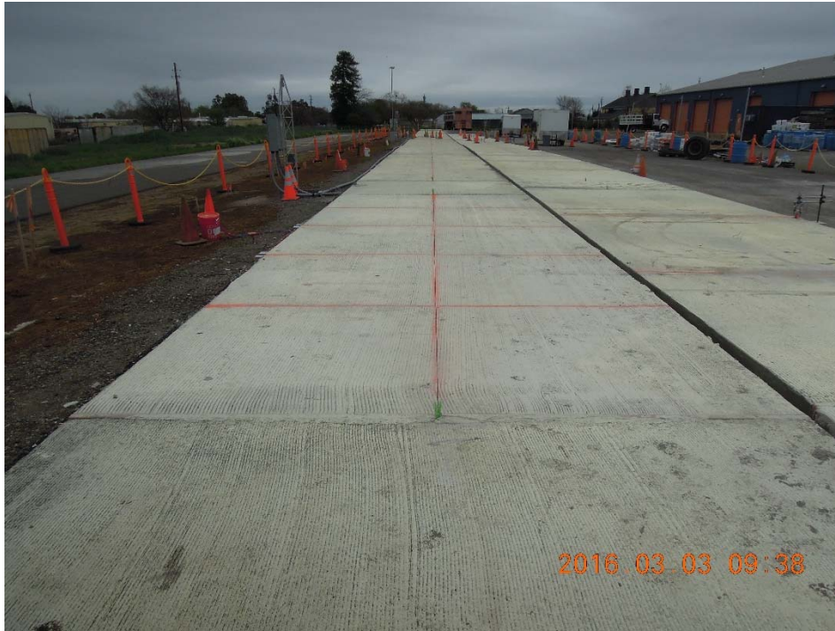
Figure A.101: Longitudinal view of test sections after paving.
