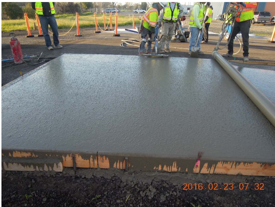
Figure A.38: Consolidation of concrete with hand-operated roller screed.
