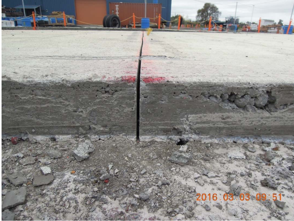
Figure A.107: Full-depth cut for separating sections.
