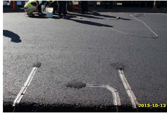
Three strain gages, after FAM protection, before extension of the RHMA-G overlay
