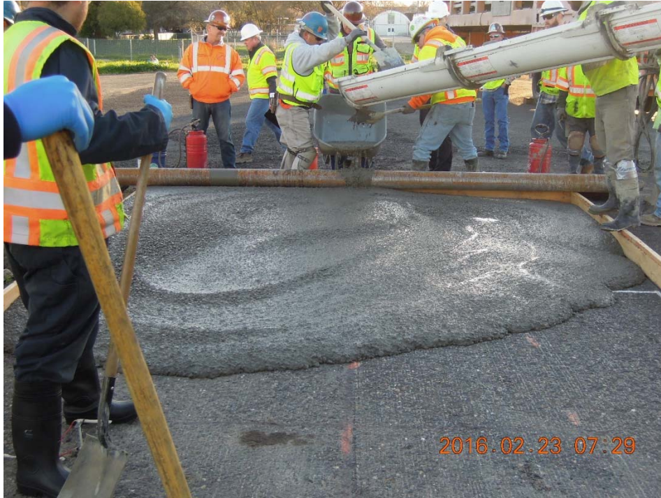
Figure A.35: Sampling of concrete for QC/QA.
