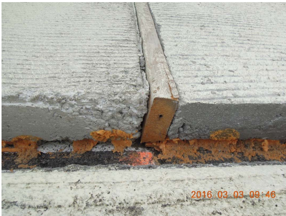
Figure A.106: Wood form for separating sections.
