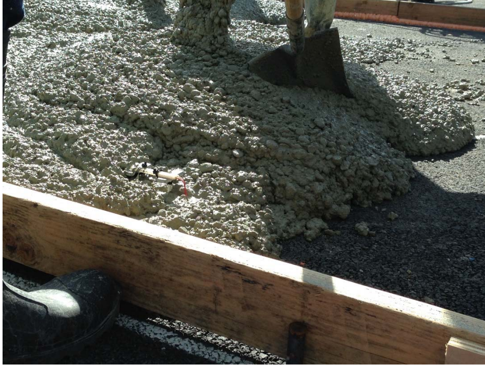
Figure A.57: Protecting instrumentation while pouring concrete.
