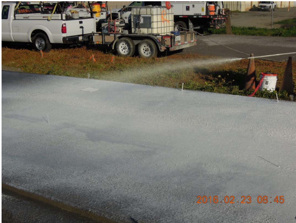
Figure A.51: Manual application of curing compound.
