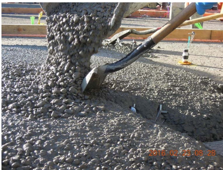
Figure 4.9: Protecting the sensors during overlay paving.
