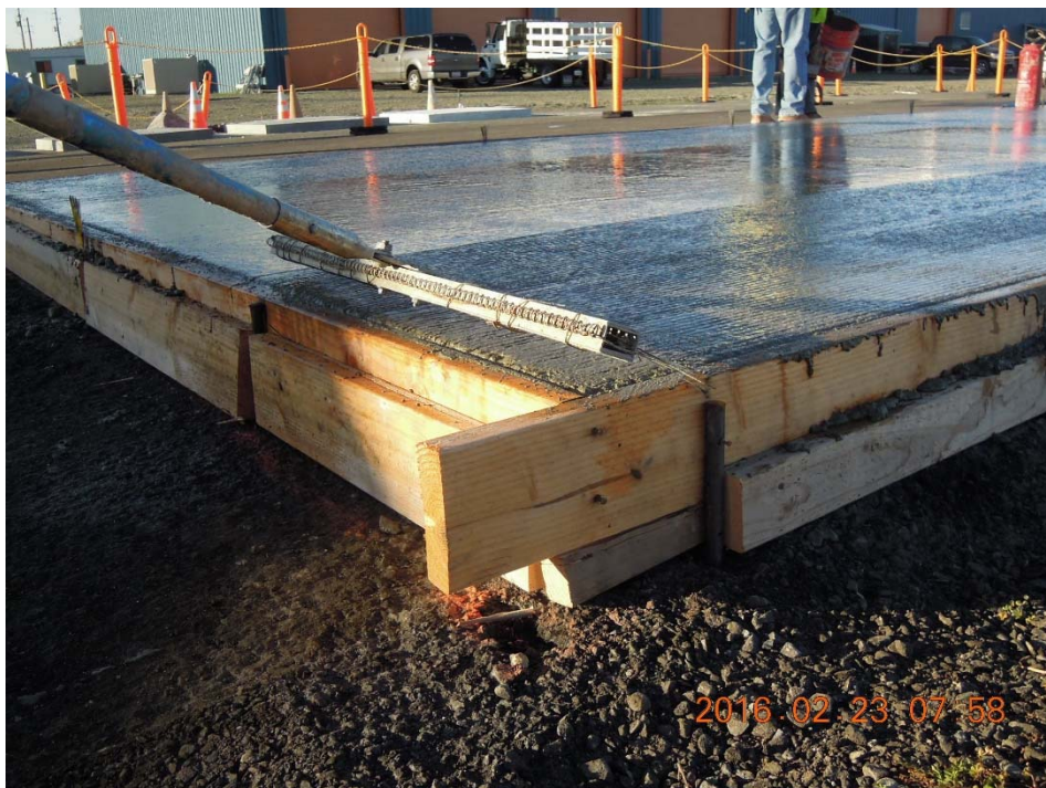
Figure A.42: Metal rake tining of the concrete surface.
