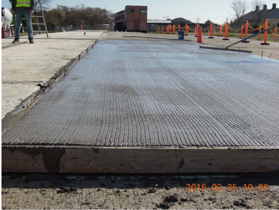
Figure A.85: Metal rake tining.
