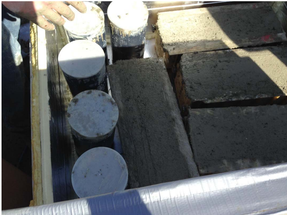
Figure A.68: Concrete cylinders and beams for QC/QA.
