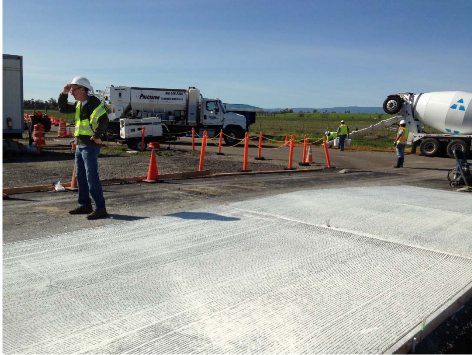
Figure A.67: Section K after tining and application of curing compound.
