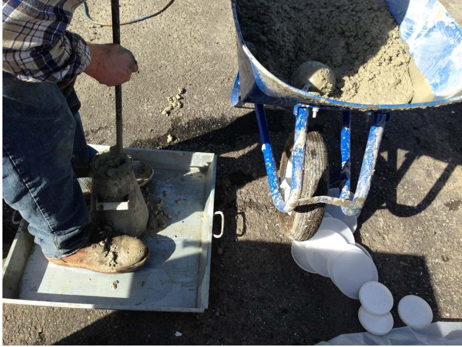
Figure A.61: Slump test.
