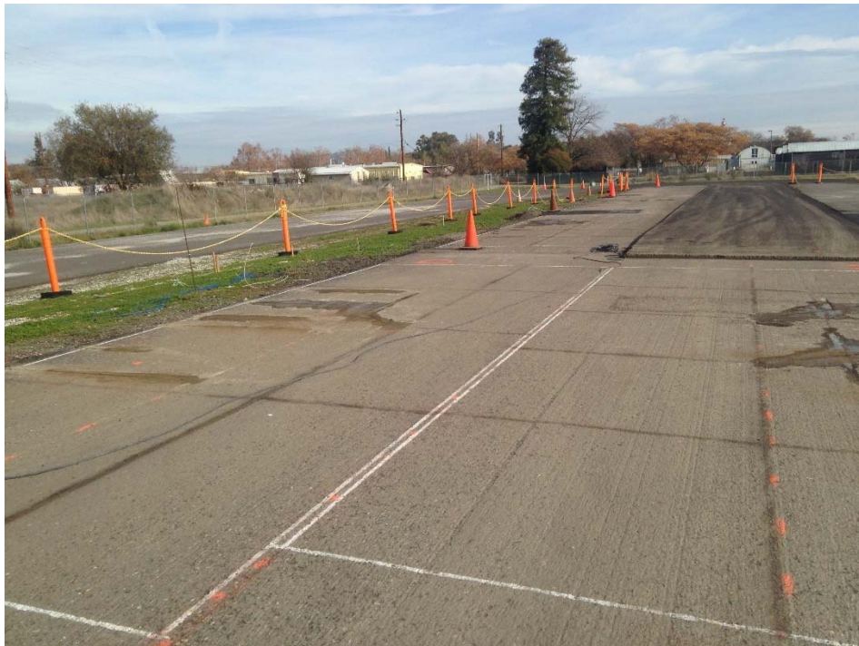
Figure A.12: Micromilled old HMA surface.
