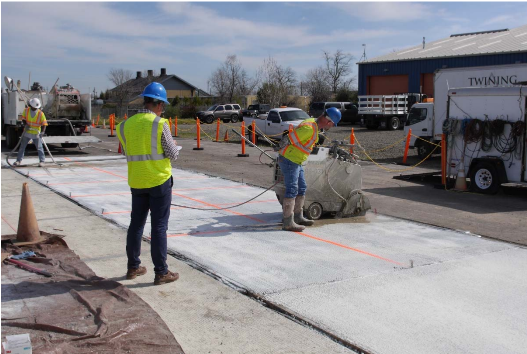
Figure A.100: Saw-cutting of transverse joints.
