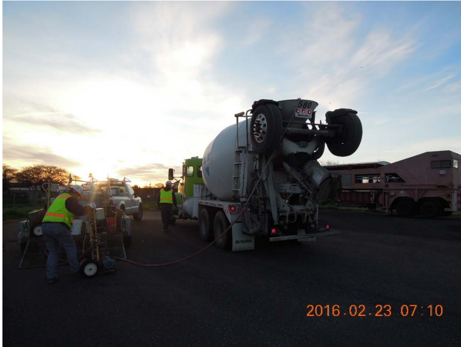
Figure A.31: First concrete ready-mix truck arriving at the construction site.
