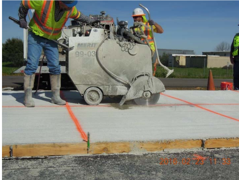
Figure 4.13: Saw-cutting operation.
