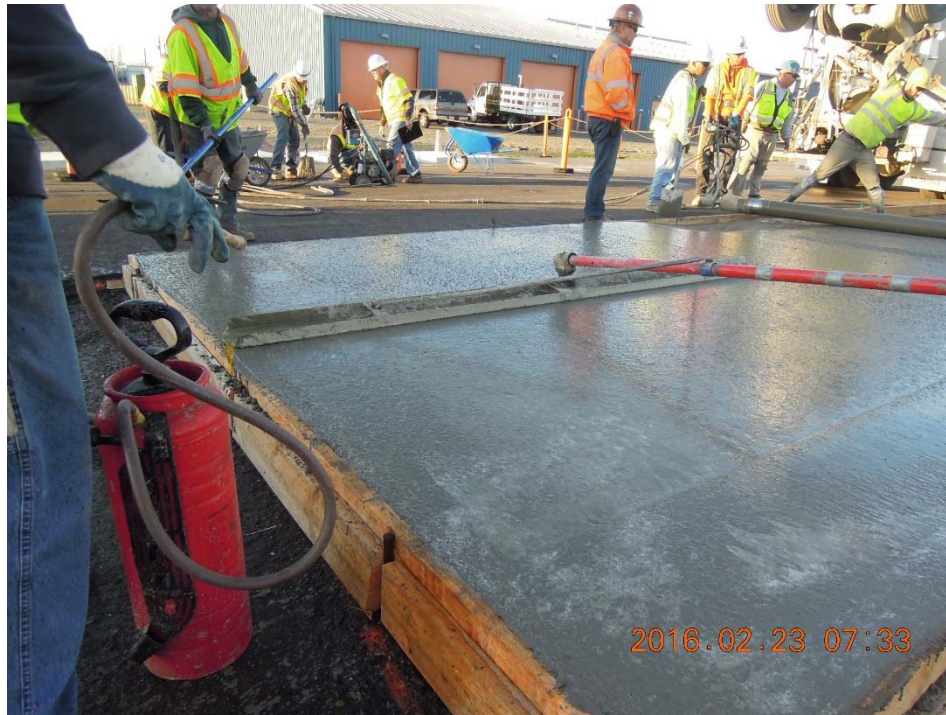
Figure A.39: Bull-float finishing of the concrete surface.
