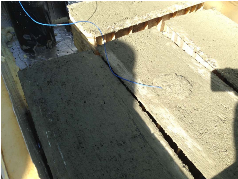
Figure A.70: A thermocouple inside a concrete beam.
