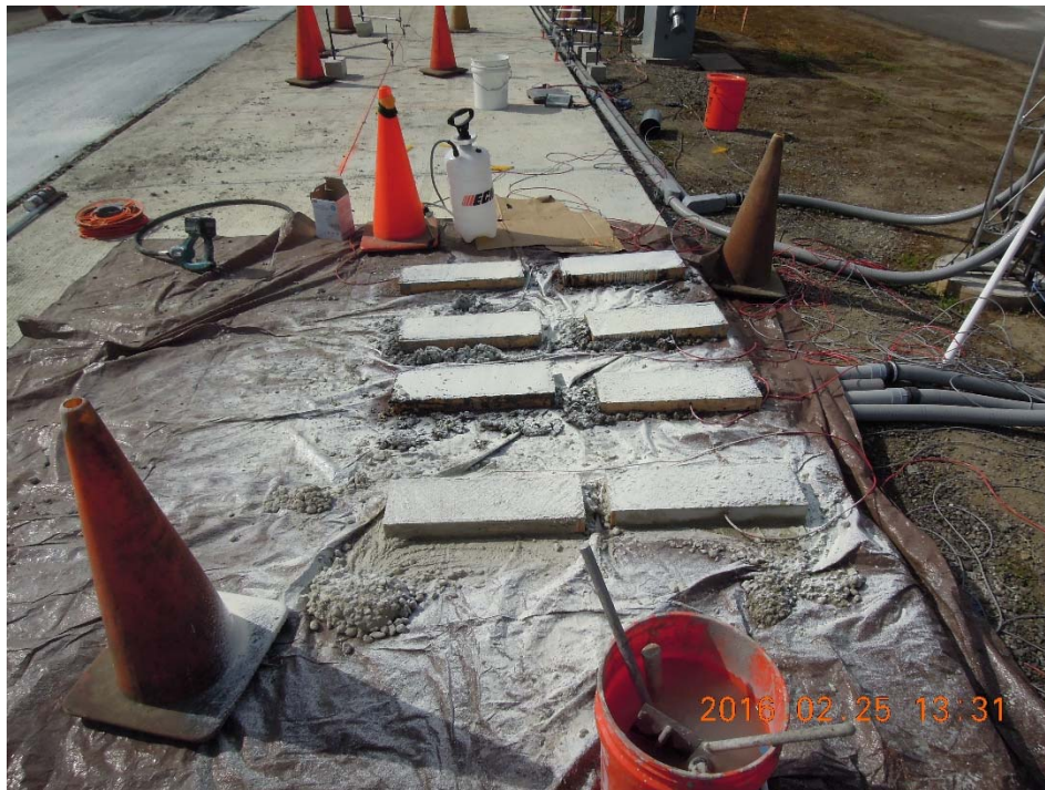
Figure A.90: Unrestrained shrinkage beams after application of curing compound.
