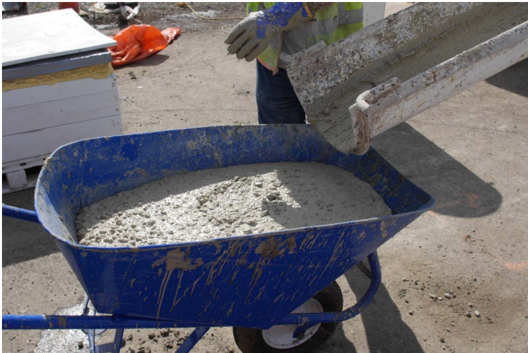
Figure A.94: Concrete sampling for preparation of specimens.
