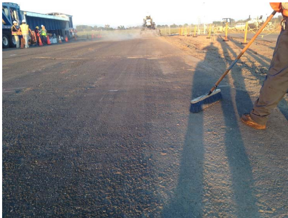
Figure A.1: Full-depth reclamation (FDR) surface cleaning and preparation prior to placement of new HMA.
