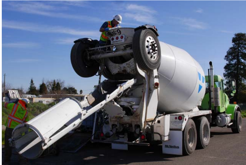
Figure 4.6: Accelerator dosed into the ready-mix truck.
