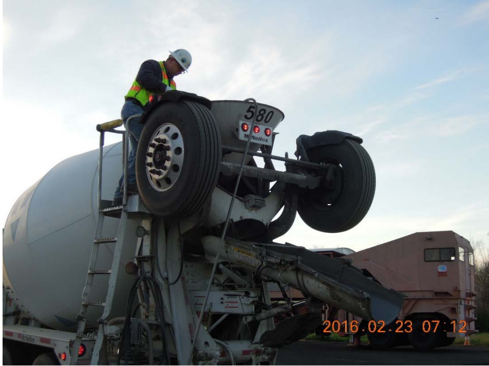
Figure A.33: Dosing accelerator into the ready-mix truck.
