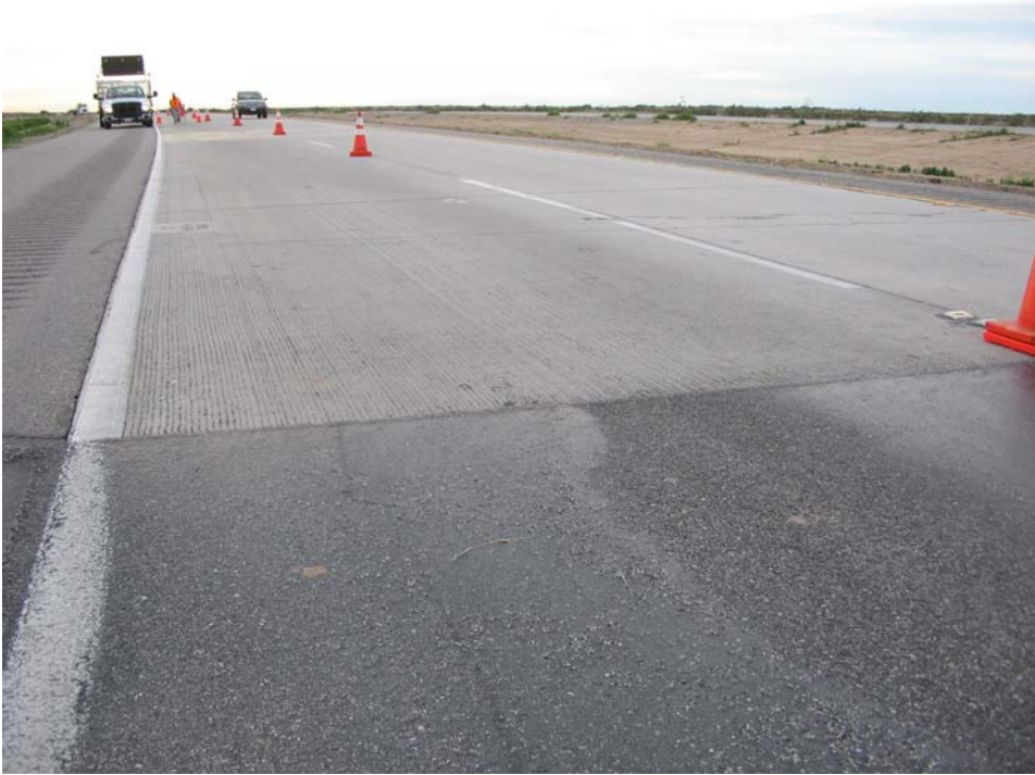
Figure 4. Station 606, facing south; RAC chip seal construction starts at this point.
