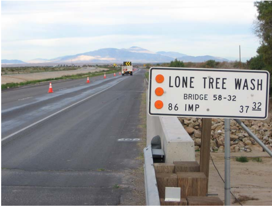
Figure 6. Station 608 (PM 37.3), facing north—flushing evident in #2 lane.
