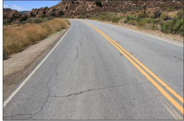
**Figure 2.4: Block crack progression.**
