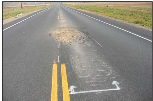
**Figure 2.6: Pumping through fatigue cracking.**
