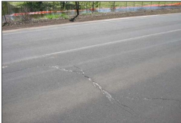
**Figure 2.1: Transverse crack.**
