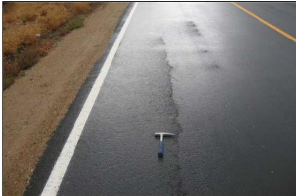
**Figure 2.2: Longitudinal crack.**
