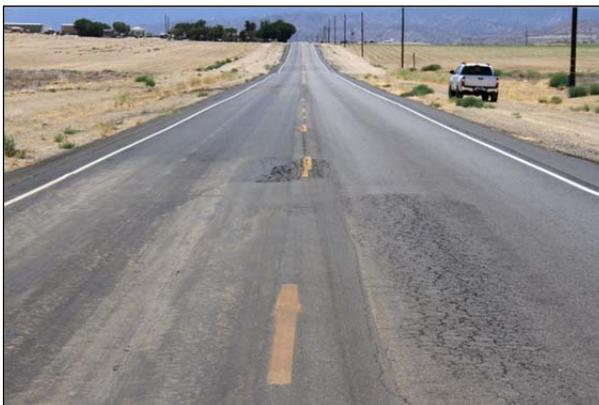
**Figure 2.5: Fatigue cracking.**
