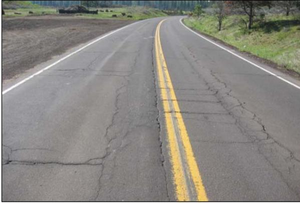
**Figure 2.3: Block cracking.**
